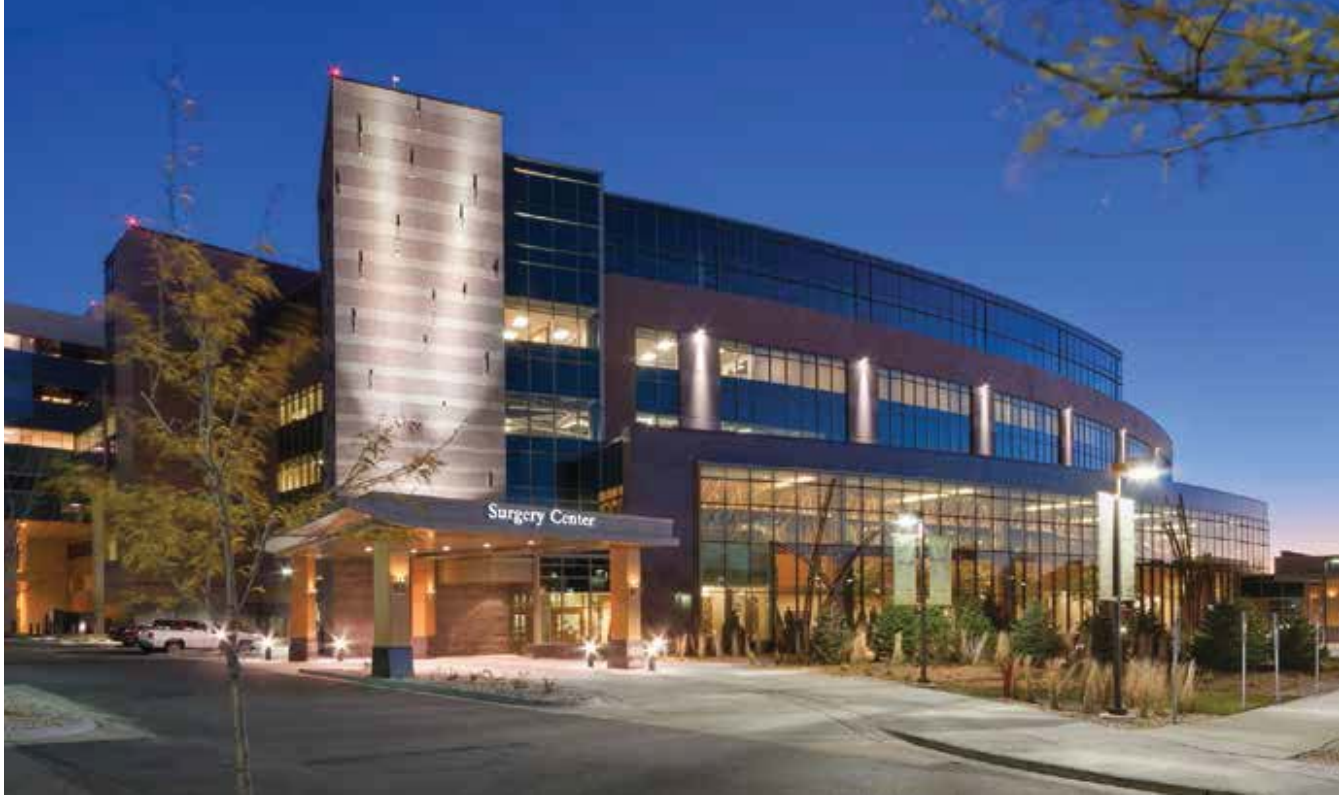
Avera Health's Prairie Center Cancer Institute in Sioux Falls, S.D., features precast concrete panels with inset thin brick, inset stone and several textures on the panels, saving more than $1 million over the original handset-brick design. Opened in 2010, the building set a new standard for the company in reducing energy consumption, using environmentally friendly construction materials, and sourcing materials locally. Gage Brothers in Sioux Falls fabricated the components. Photo: Avera Health.
