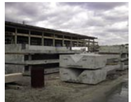
Fig. 13. Stair-stepped column covers were integral to establishing the historic, traditional ambience desired by the owner. (Courtesy of Metromont Corporation)
