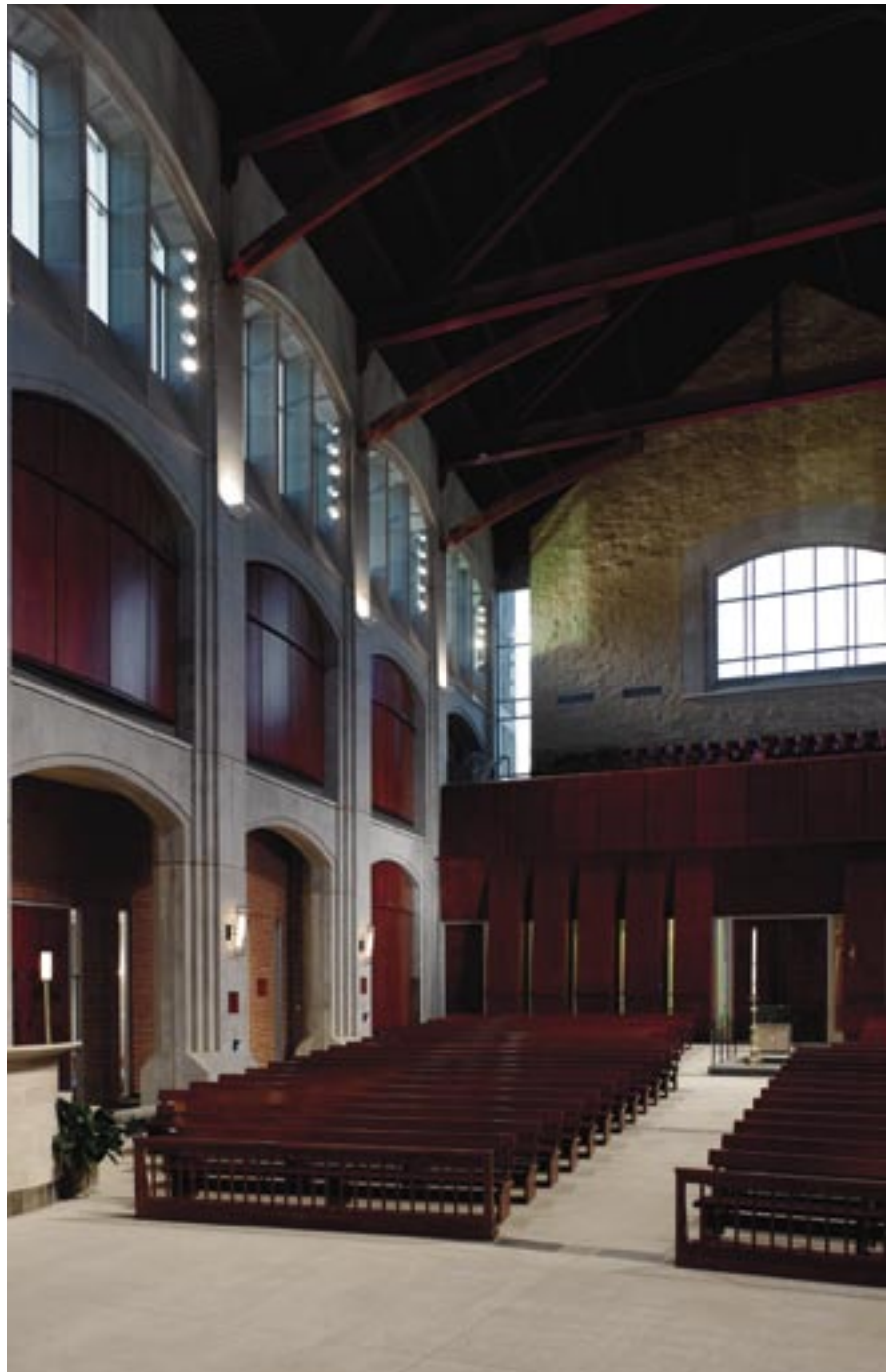
Fig. 5. Precast concrete arches emulate the traditional architecture of historic worship spaces and simultaneously create the modern aesthetic of natural stone. (Courtesy of Brian Dressler)
