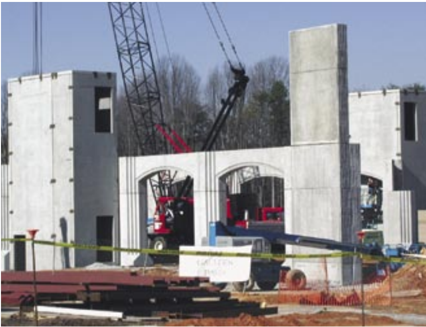
Fig. 10. Erection of the first precast concrete walls. (Courtesy of Don Brown, Metromont Corporation)
