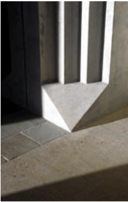
Fig. 18. Close-up view of foot of column in the narthex. Precast concrete is particularly effective as a foil to the slate and salt-finished concrete floor. (Courtesy of Brian Dressler)
