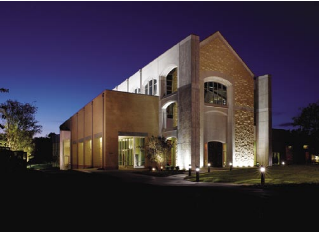
Fig. 20. Taken at night, this photo of the completed Prince of Peace Catholic Church highlights the striking and appealing look of natural stone created with a precast concrete architectural finish. (Courtesy of Brian Dressler)
