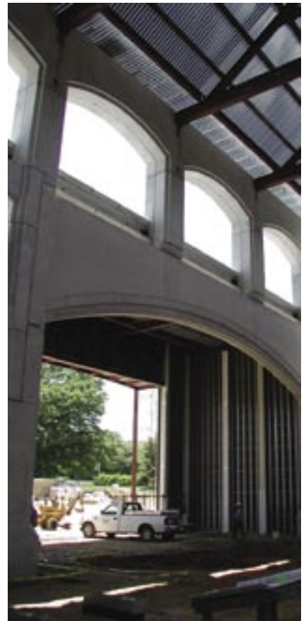
Fig. 12. An interior view showing the precast concrete arch in position. (Courtesy of Randy Davis, Design/Build Engineers, Inc.)
