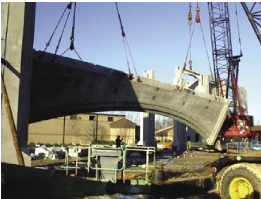
Fig. 11. Two cranes hoisting the 77,000 lb (35000 kg) precast arched spandrels. Note the special rigging with numerous pick points. (Courtesy of Jeff Hargett, Metromont Corporation)
