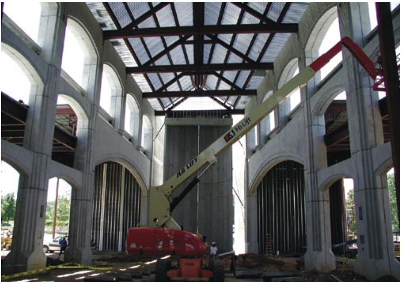
Fig. 7. Steel roof trusses bearing on precast concrete walls required careful attention to detail, as the precast concrete walls were not parallel. (Courtesy of Design/Build Engineers, Inc.)
