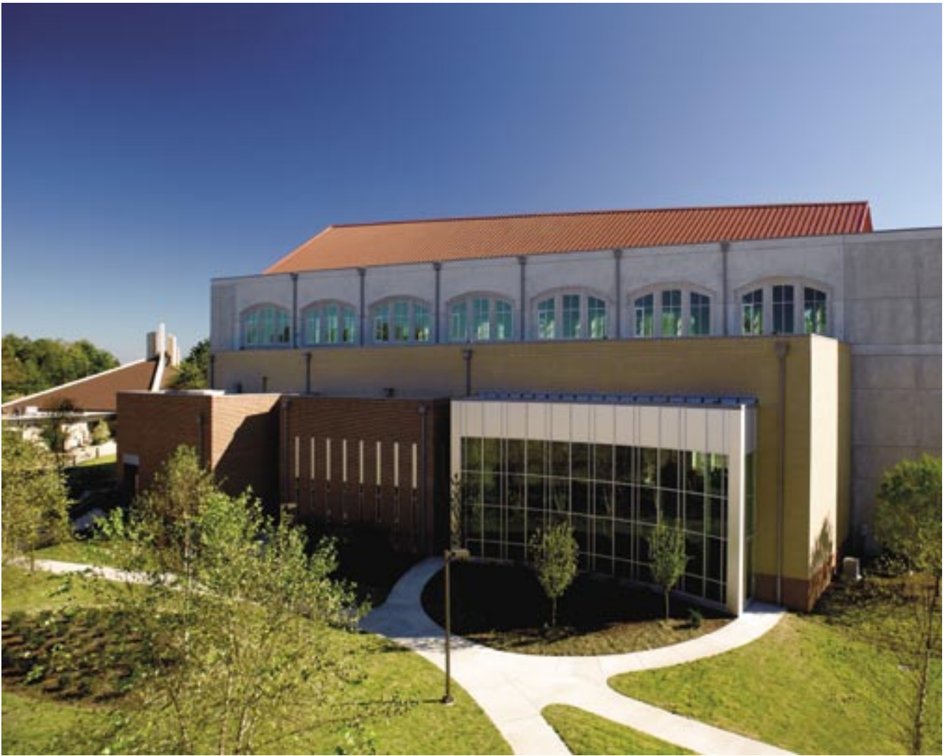
Fig. 9. A landscaped interior walkway offers communicants a preparatory environment distinct from street and parking areas. Note the original 1965 steel-frame structure in the background to the left. (Courtesy of Brian Dressler)
