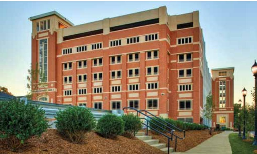
The new eight-level, 1,002-car parking structure at Central Piedmont Community College features a total-precaster concrete structural solution. Two concrete pigments, one between bricks and one on larger portions, sometimes in the same panels, were used to achieve the appearance that the designers sought.
