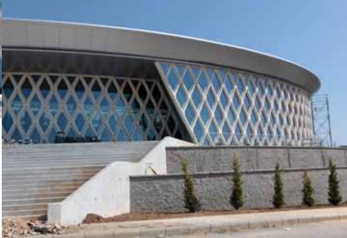
*The new Nanotechnology Research & Application Center at Sabanc University in Turkey features an innovative use of precast concrete as a structural lattice that symbolizes the work accomplished at the facility. The precast concrete lattice consists of 53 modules, each 24 feet high and 20 inches thick, with a layer of insulation sandwiched between two layers of concrete.*
