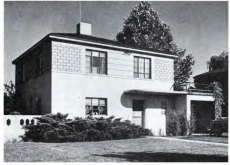
Fig. 3B. Two-story precast concrete house in Silver Spring, Maryland, built in 1935 by the Earley Studio (Courtesy: Joseph W. Molitor).
