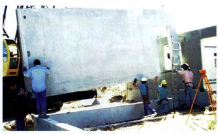
Fig. 9B. Workers guide panel into position on precast foundation wall.
