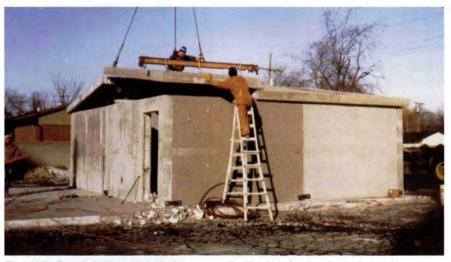
Fig. 10A. Prototype structure being erected with site-cast laminated panels. Precast panel used for sloping roof.
