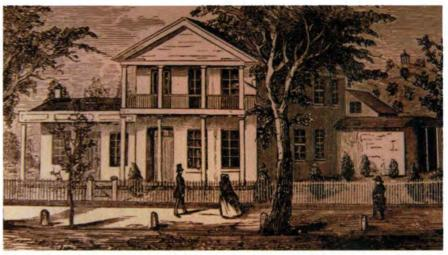
Fig. 1. *The Poor Man's Home and the Rich Man's Palace* was the title of a book George Barrett published in 1854 to describe construction of this concrete house in Spring Valley, Ohio. The sand, gravel, and lime mix was supplemented in some places with cobblestones to speed filling of the forms.
