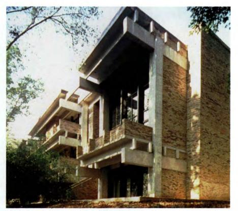
Fig. 6. This prestigious, custom built home was built with precast, prestressed concrete in mind from the outset. Columns, beams, double tees and lintels framed the house. The project won a PCI Award in 1987. Reference: PCI JOURNAL, September-October 1987, p. 27. (Continued on p. 66)
