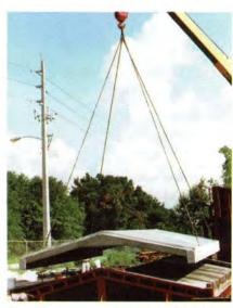
Fig. 7C. Precast concrete roof module being lifted from its form.
