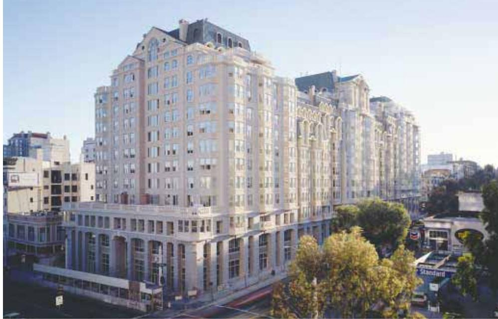
*San Francisco Towers is a life care community utilizing the light weight and aesthetic range of glass fiber reinforced concrete (GFRC) in a high seismic zone.*
