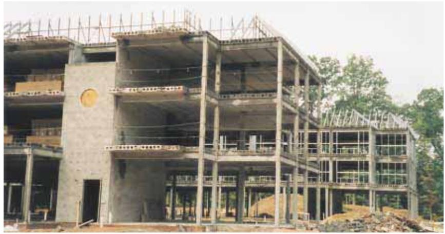
Hollowcore helped the Marriott meet restrictions on building height, providing a tall floor-to-ceiling room space on each level. Mechanical and electrical needs were run through the cores in the slabs to facilitate using the plank as a combined ceiling/floor.
