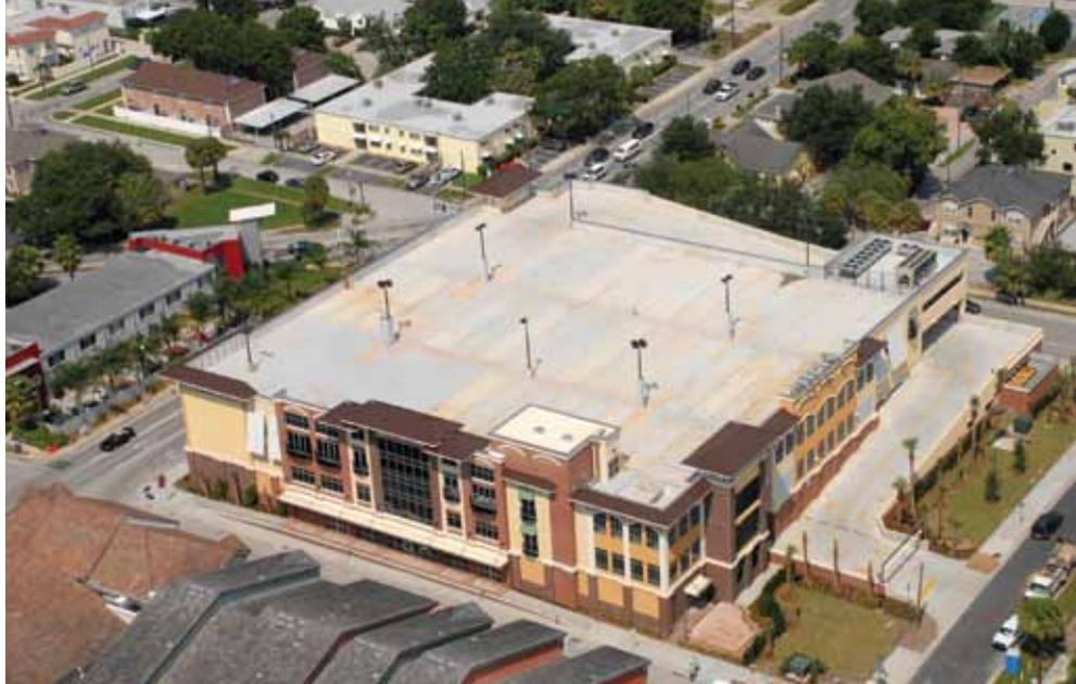
*The tight site required the structure to be built from the inside out, positioning the crane inside the footprint and working across the building before backing up to erect the next set of bays. When the crane finished the final portion, the speed ramp to the parking levels was built as the final piece.*
