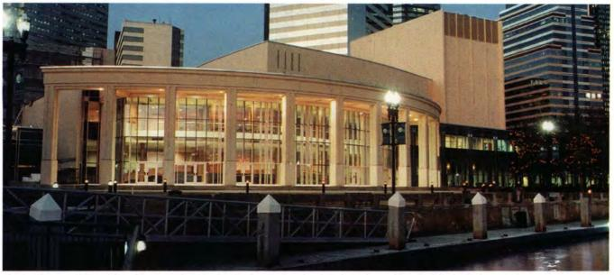
Fig. 1. The new \$32 million Times-Union Center for the Performing Arts in Jacksonville, Florida, includes a \$10.6 million concert hall (foreground) consisting of an all-precast concrete structure, including loadbearing acoustical walls for the theater.
