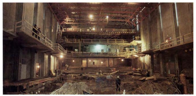
Fig. 8. Using precast concrete panels allowed the new theater to be enclosed much faster than would have been possible with other systems. It also provided the strength and thin profiles required to add two balconies into the space and reach the necessary seating requirement.
