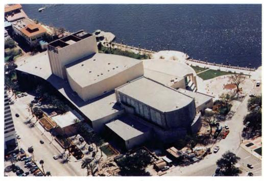
Fig. 2. Aerial view showing how the new theater (foreground) attaches to the existing two other theater sections in the building. The rear wall was removed and extended to accommodate the new three-level theater.
