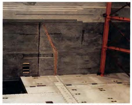
Fig. 14. The balcony slabs were cantilevered and connected to the back wall of the theater, which was also made of precast concrete.
