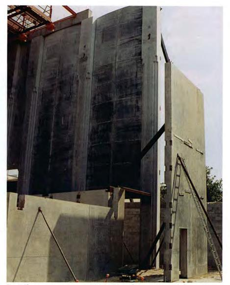
Fig. 9. The precast structure comprises a variety of components, including loadbearing panels that were curved on the interior for proper acoustics and flat on the exterior. These exterior walls were furred out and clad with drywall to serve as the corridor outside the theater.
