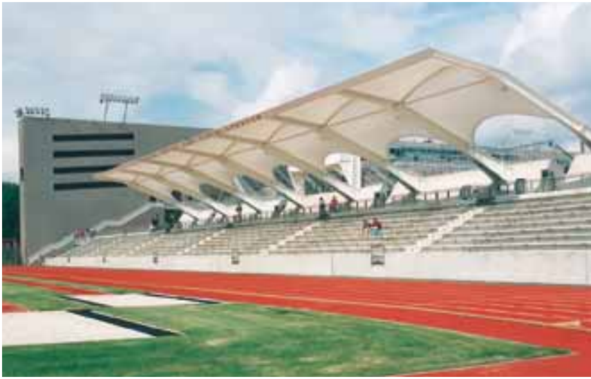
The adjoining track stadium features precast concrete seating covered with a fabric canopy held in place by cantilevered steel posts. The units are monolithic with precast concrete seating facing the other direction to enclose the open end of the football field's seating. Photo: Paul Warbcol Photography Inc.
