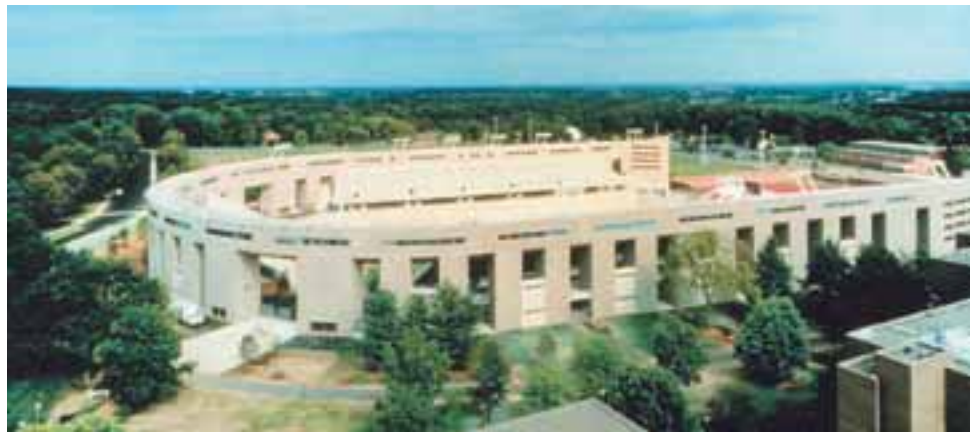
This overview shows how the horseshoe-shaped stadium connects visually to the track stadium at its open end and further along to the 1960s gymnasium at the far right. Photo: Paul Warbcol Photography Inc.
