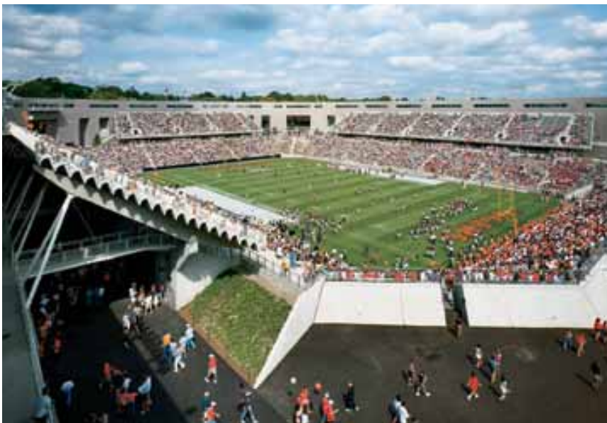
Princeton University’s new stadium features several unique aspects. These include the trapezoidal upper seating on three sides, made of precast concrete triple risers, and a perimeter building housing all services that remains open year-round, as does the colonnade behind the seating sections. Photo: Chuck Choi, ESTO
