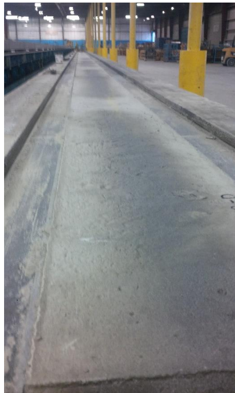
Figure 3: Ties in a long-line bed form
