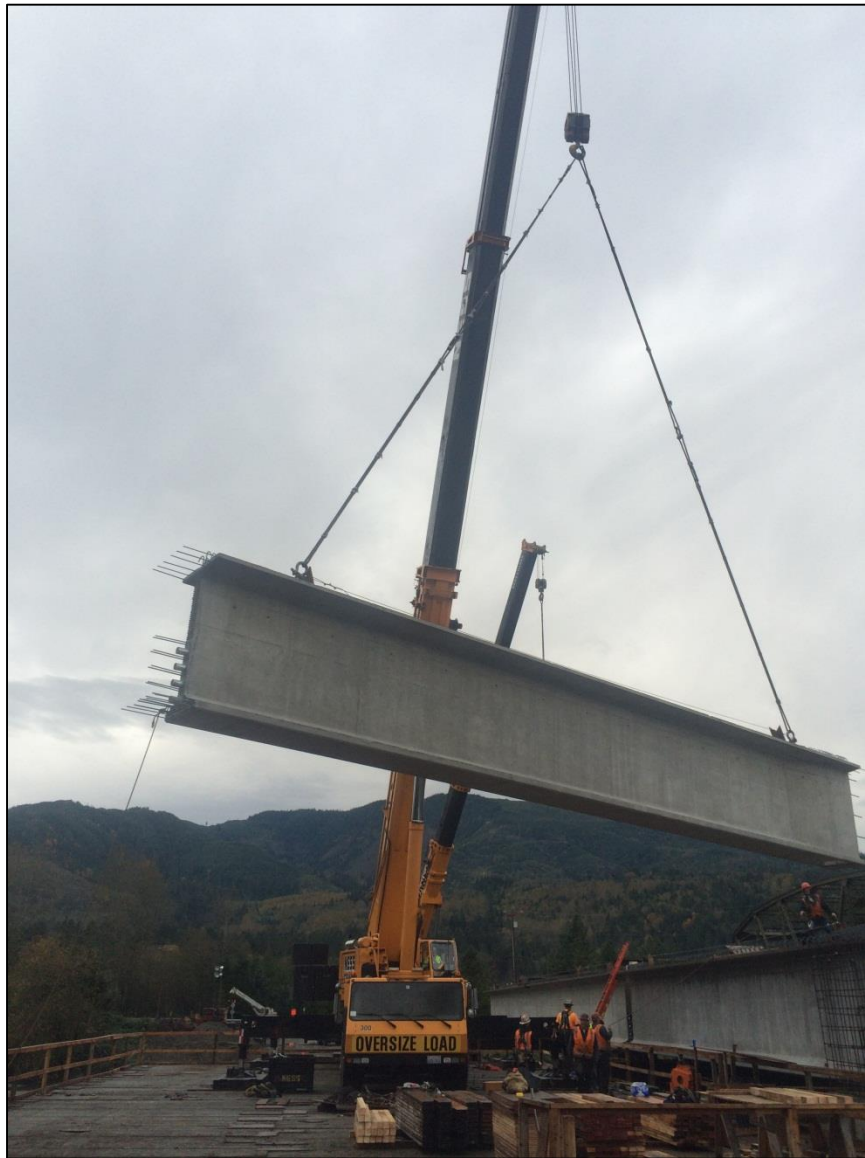
Fig. 5 On-Site Erection of Post-Tensioned Spliced Girder Segment 3 Girder Segment
