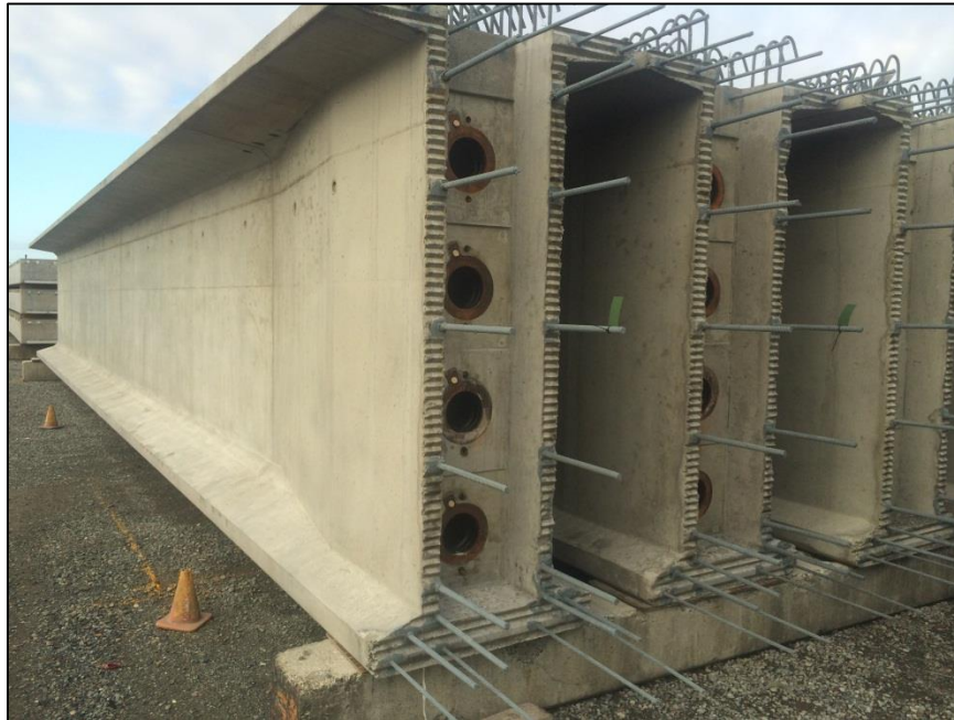
Fig. 4 Stored Post-Tensioned Spliced Girder Segment 3 Girder Segment
