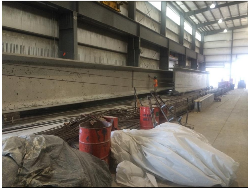
Fig. 6 Casting of Segment 2 Girder Segments
