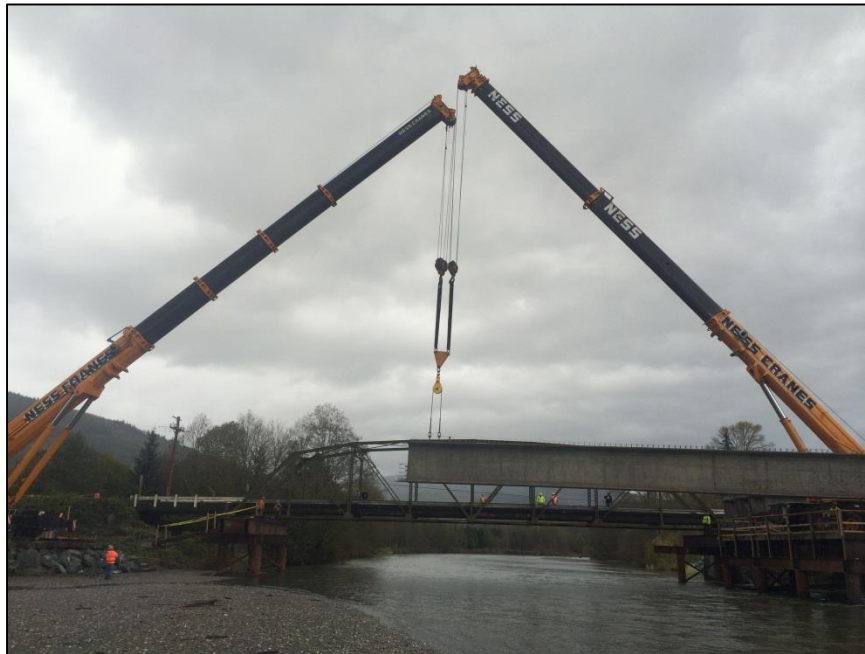
Fig. 9 Transfer of the West End of Segment 2 Girder Segment
