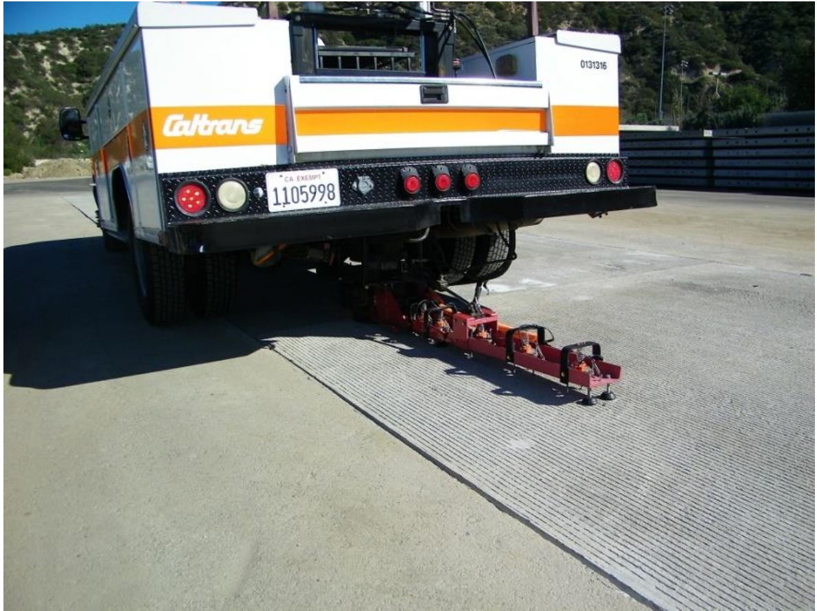
Fig. 5 Evaluation of Load Transfer Efficiency Using FWD for a Proposed New System
