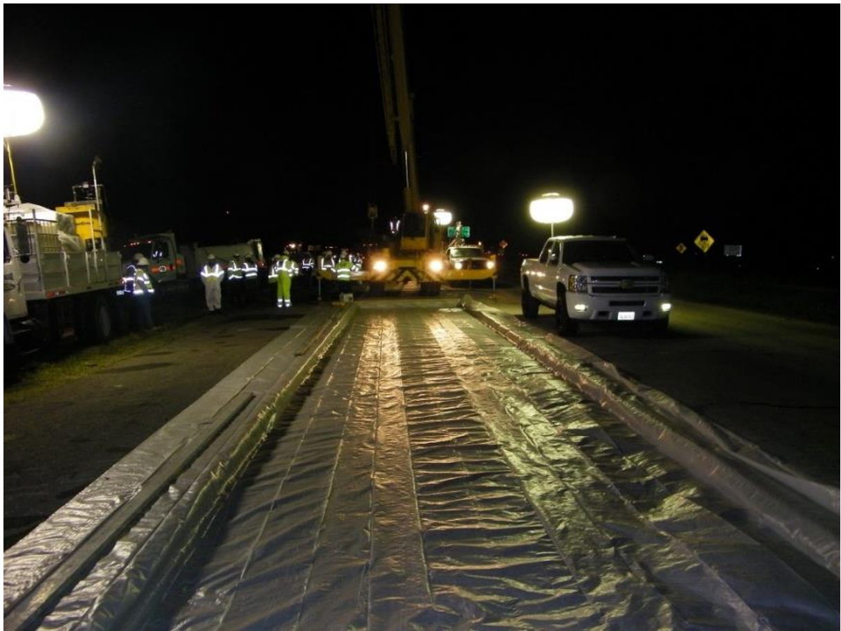
Fig. 7 Use of a Polyethylene Sheet under the Panels for a PJCP Job
