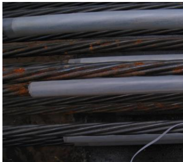
Fig. 2 Plastic sheathing used for debonding strands
