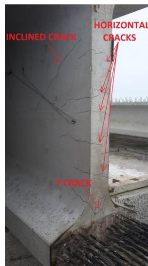
Fig. 1 Types of prestressed concrete girder end cracks
