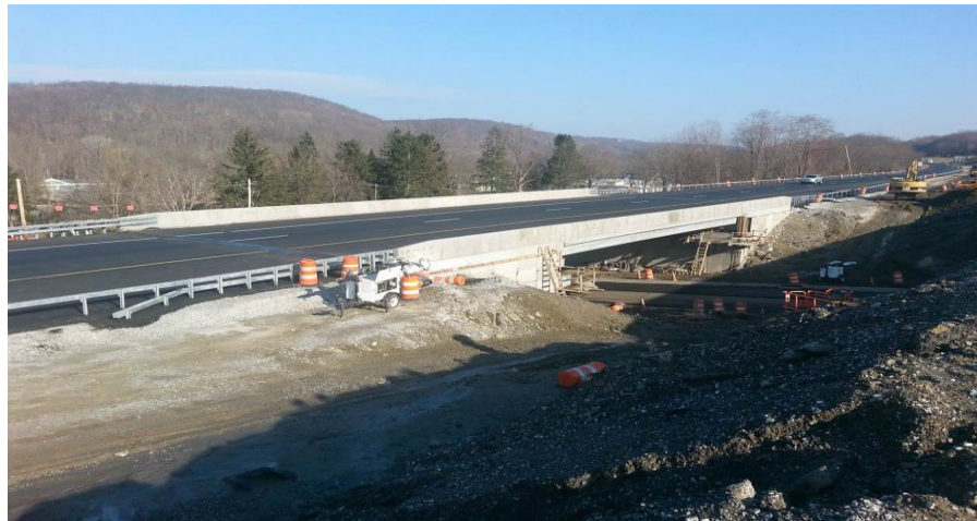
Figure #6 – Second Bridge Open to Traffic
