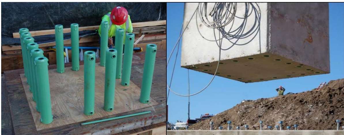
Figure 1 – Grouted Bar Splicers
