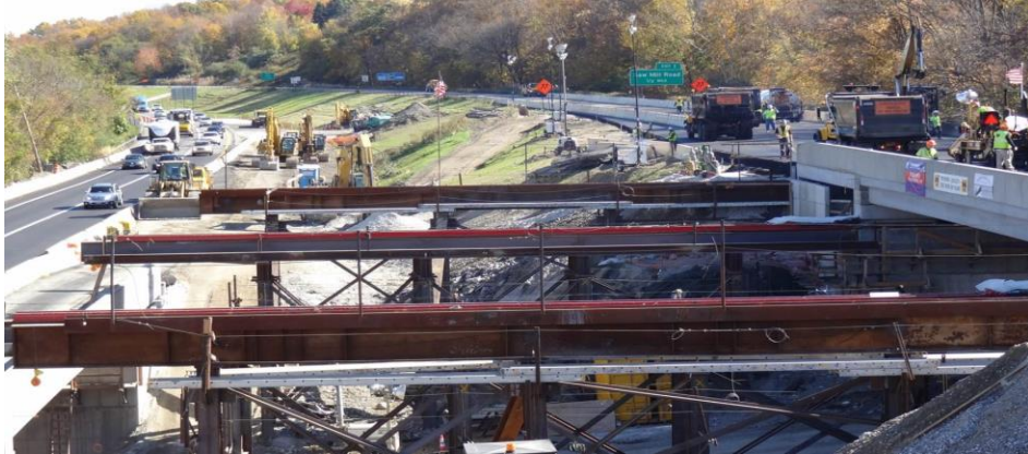
Figure #5 – First Bridge Moving Into Position
