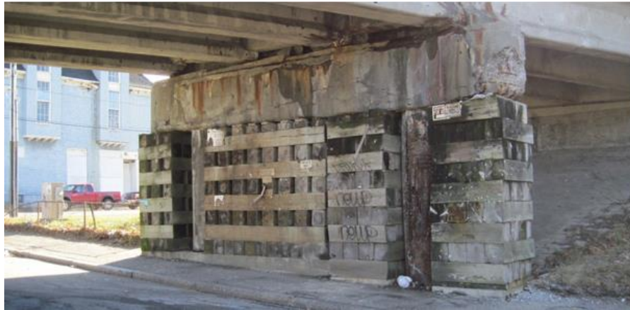
Figure 7 – Existing Bridge Conditions
