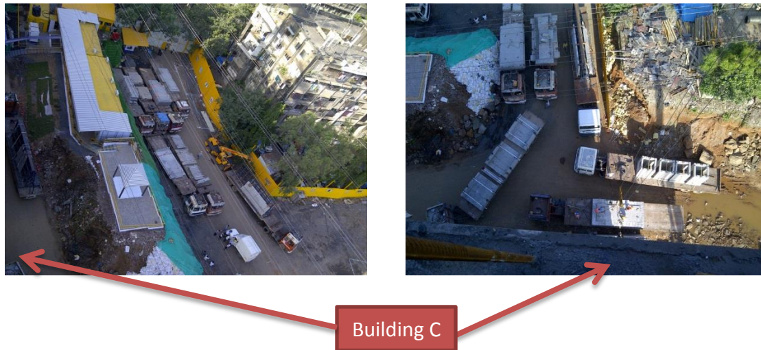
Fig. 11 Pragati Towers – Phase 1 Site
