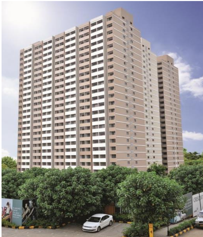
Fig. 3 Completed Towers (Part 1 of Phase 1)
