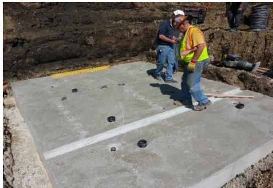
Fig. 12 Finishing the erection of the base slab
