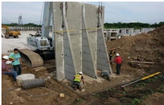
Fig. 13 Final assembly of TPCCRW
