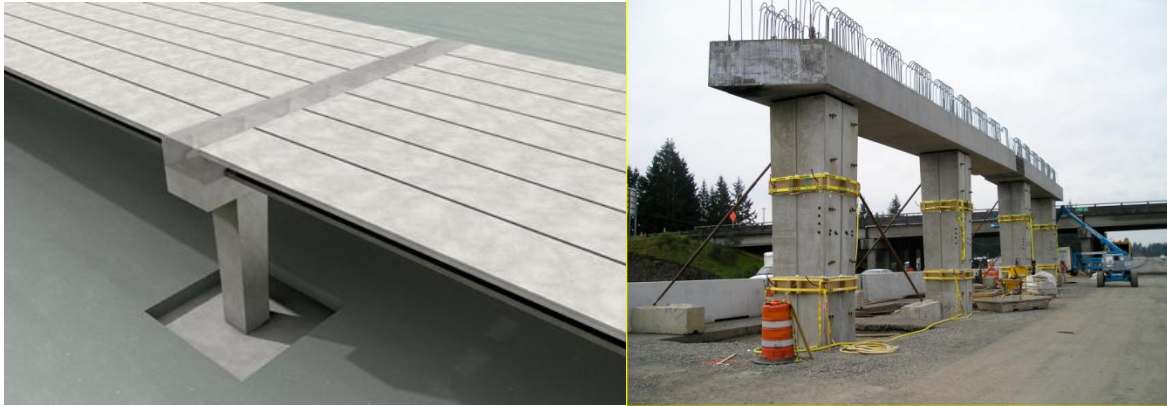
Figure 4. Semi-raised fixed integral diaphragm
