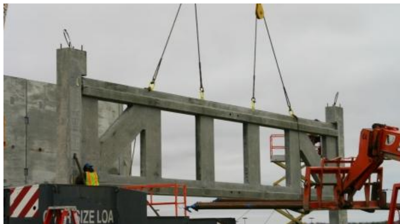
Fig. 3 Erection of ER-POST trusses [6]
