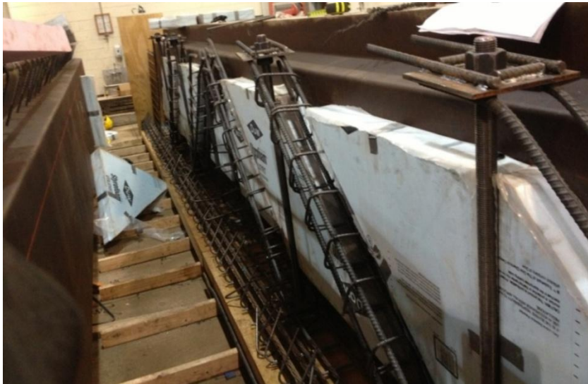
Fig. 15 Form block-out and vertical and diagonal reinforcements
