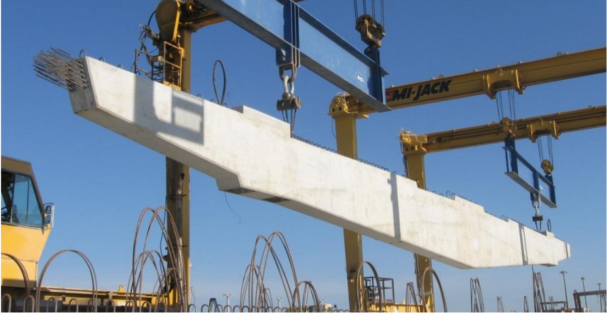
Fig. 10. Lifting Precast Floor Beam from Casting Bed
