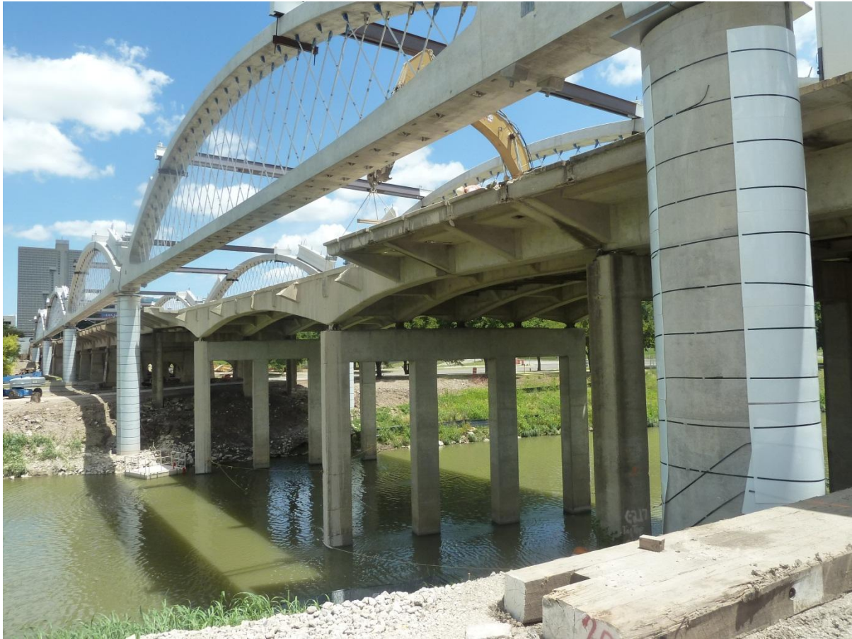
Fig. 3. 7'-3" x 5'-6" Oval Columns and Demolition of Old Bridge
