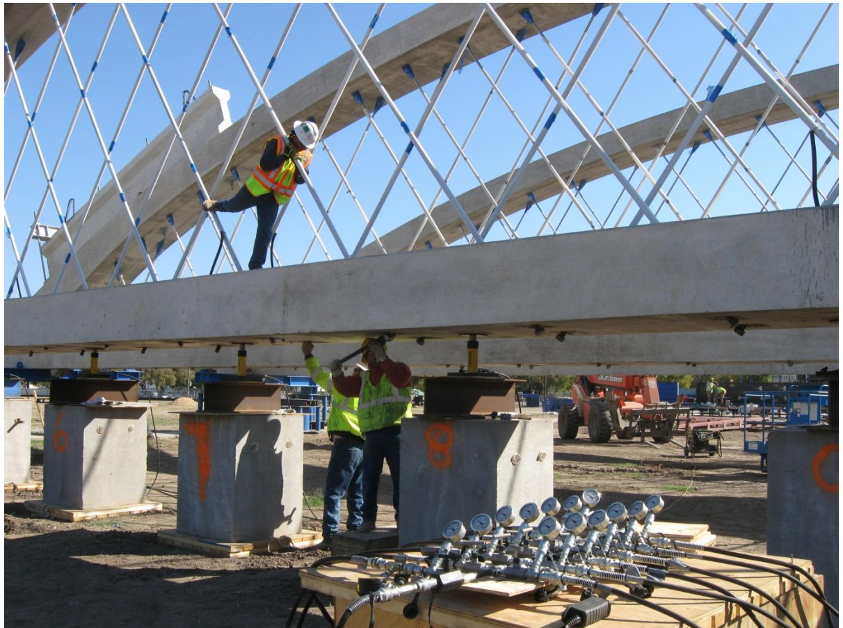
Fig. 6. Lifting the Arch Tie with Hydraulic Rams and Tightening Hanger Nuts
