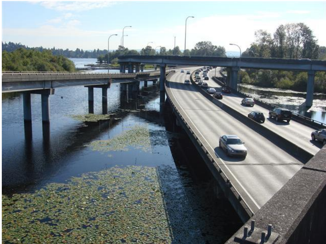
Fig.1 Existing bridge to be widened, lower bridge
