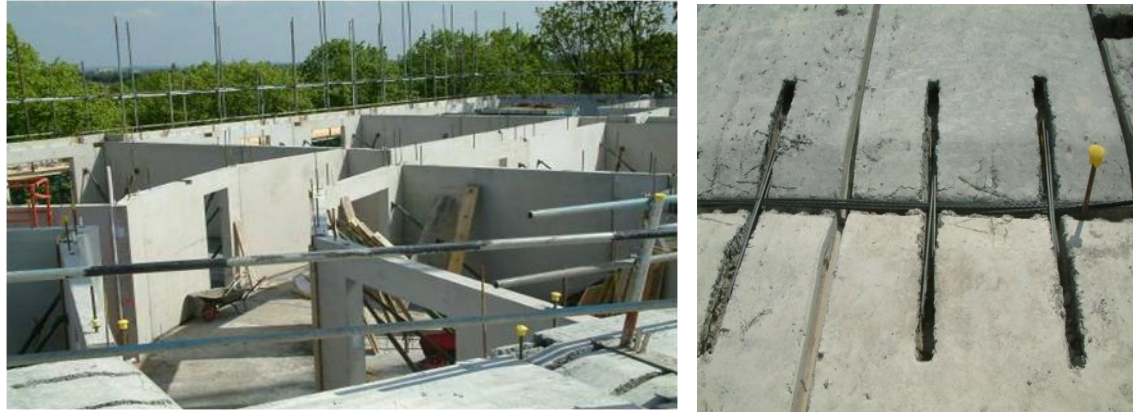
(c) Precast cross wall structure
