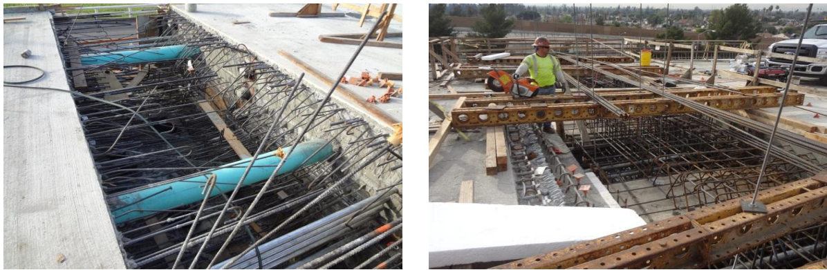
Fig. 1 In-span hinges in CIP/PS box girder bridges
