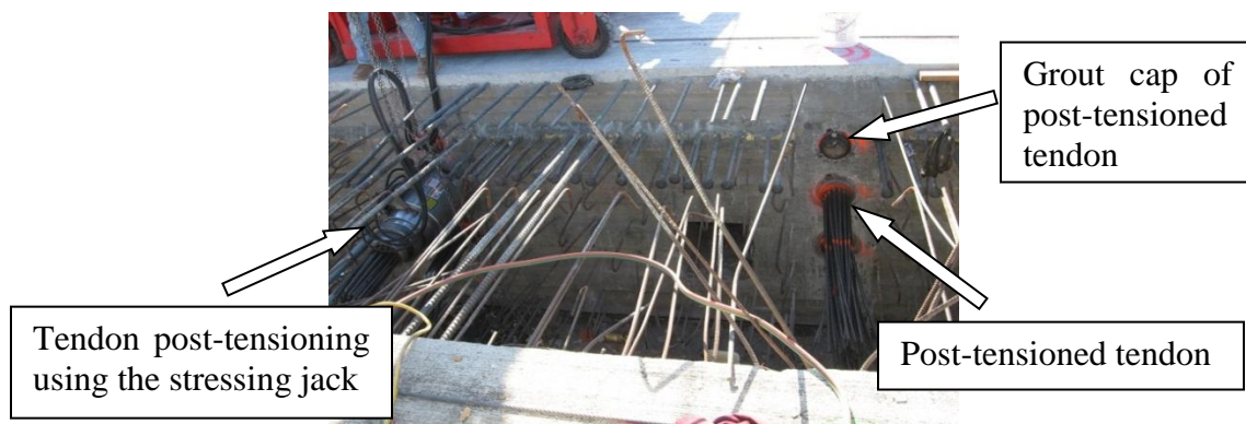
Fig. 3 Post-tensioning process at hinge 7 (San Luis Rey River Bridge)
