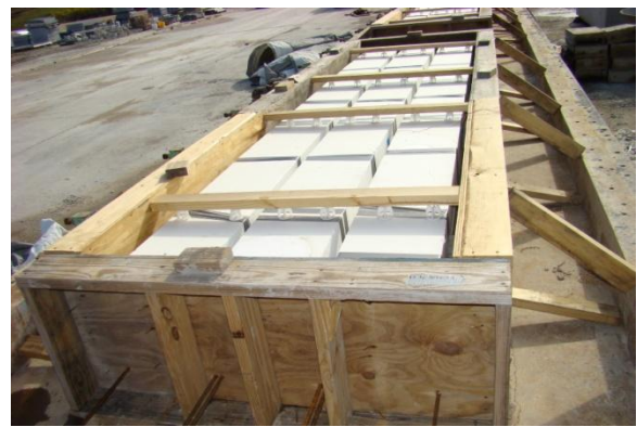
(b) Preparation of formwork
