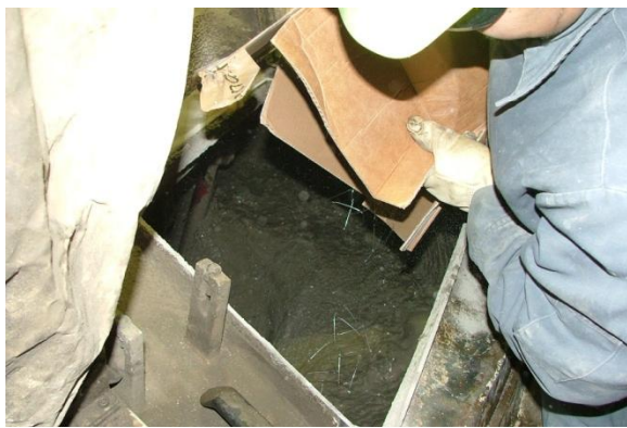
(a) Concrete mixing with steel fiber
