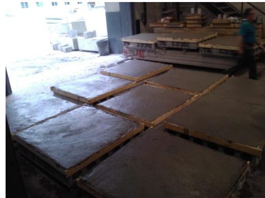
(b) After casting the topping
