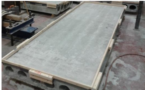
(a) Before casting the topping
