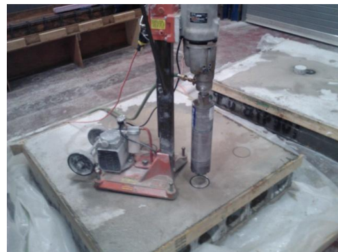
(b) Drilling process
