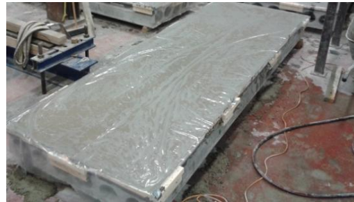
(b) After casting the topping
