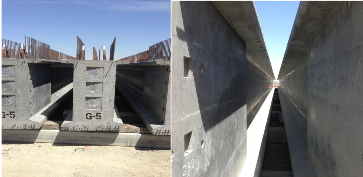
Fig. 6 - Post-Tensioned Wide Flange Girders fabricated for Riego Road OC
