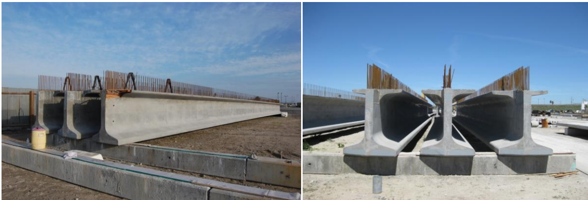
Fig. 5 - Pretensioned Wide Flange Girder fabricated for Butterfield Blvd
