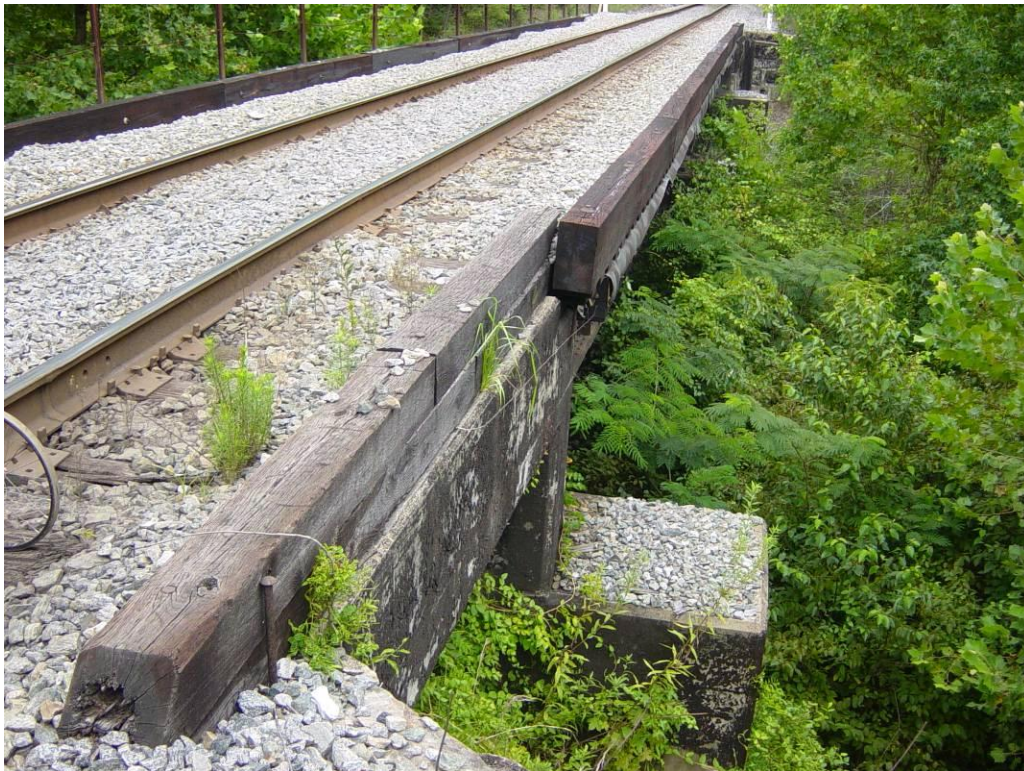
Fig. 9, Project Site Prior to Construction
