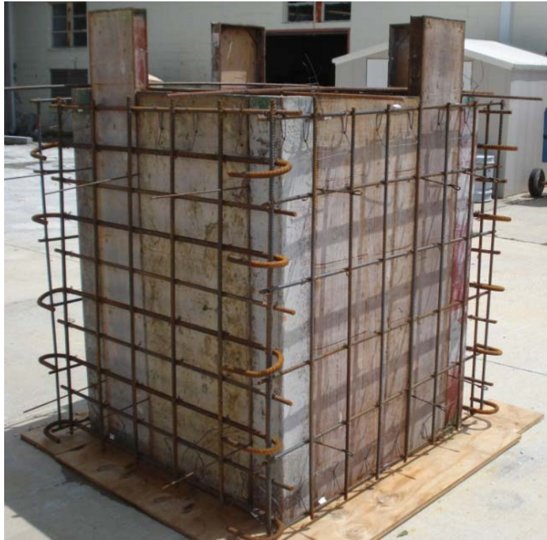
Fig. 3 Box culvert and reinforcing steel.
