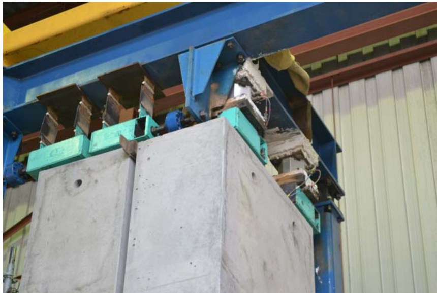
Figure 8. Seismic Joint at Corner Assembly (vertical seismic joint between panels will close when the return panel moves in the U1 direction)
