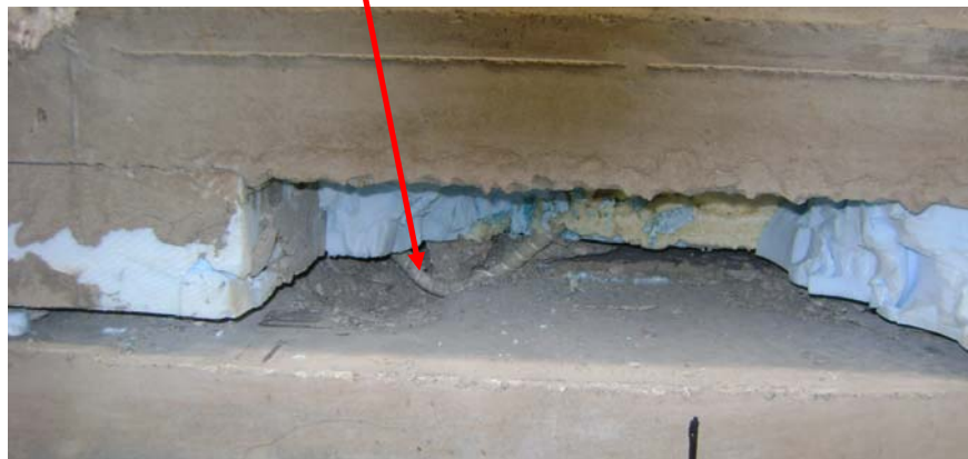
Figure 10: Pull out of GFRP tie at failure
