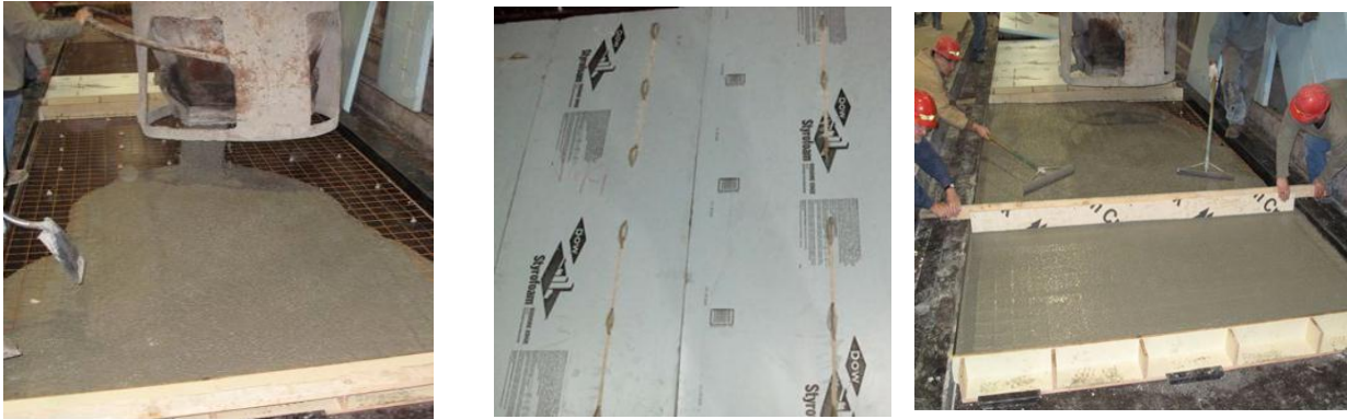
Figure 5: Fabrication sequence of PCSPS A and B
