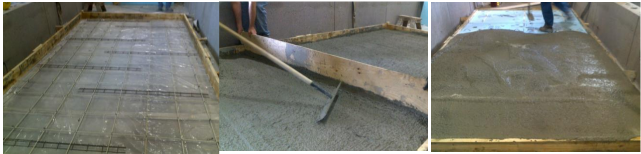
Figure 6: Fabrication sequence of PCSP C
