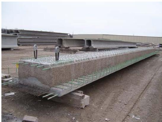
Fig. 13. (a) Completed Interior Beam
