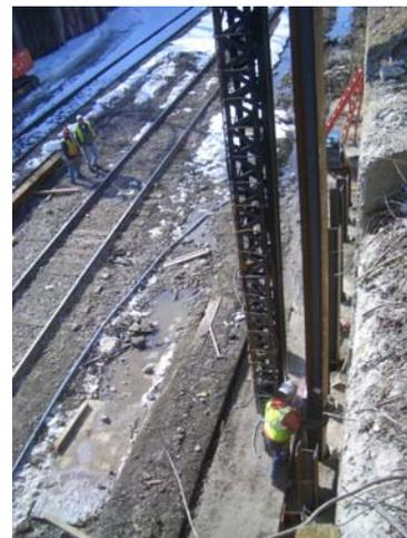
Fig. 8. (a) Holes Drilled in Existing Abutment Toe
