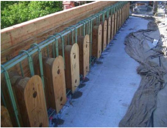
Fig. 17. (a) Forming Parapets
