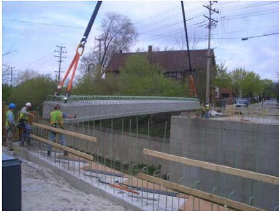
Fig. 14. (a) First Exterior Beam
