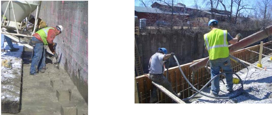
Fig. 9. (a) Holes with Grout
