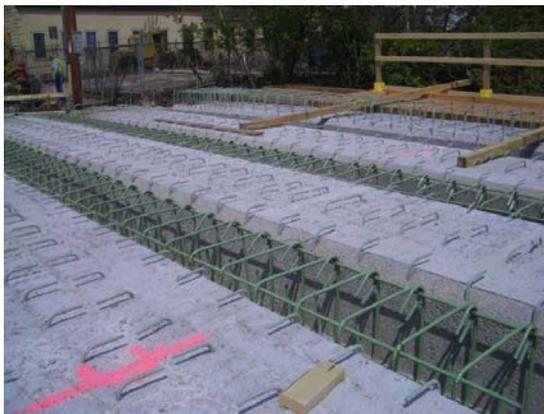
Fig. 16. (a) Slab Re-bar Cages Installed
