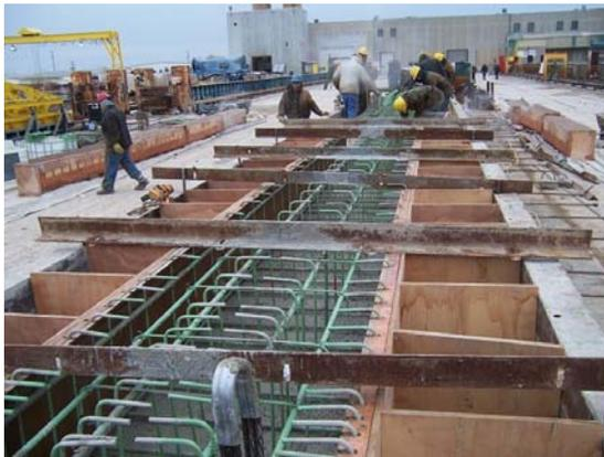
Fig. 12. (a) Forming Interior Beam
