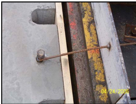
Fig. 13 - Shear Connector Half Blockout (Mosquito Bridge)
