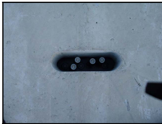
Fig. 14 - Shear Connector Blockout (Haverhill-Newbury)
