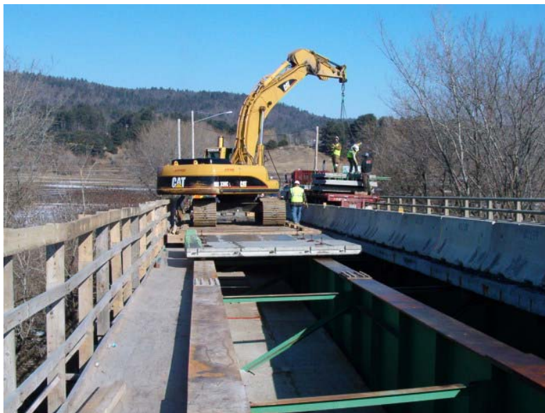
Fig. 8 Placement of Deck Panels
