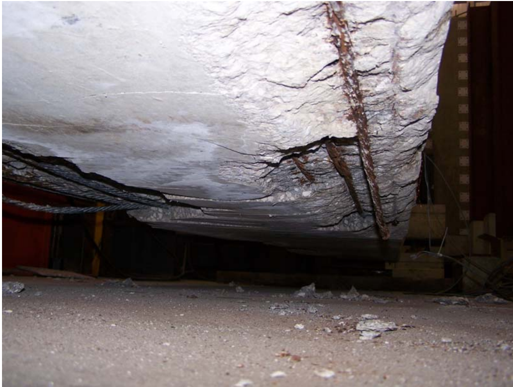
Fig. 14: Destructive Test of Beam 16 (Bottom)
