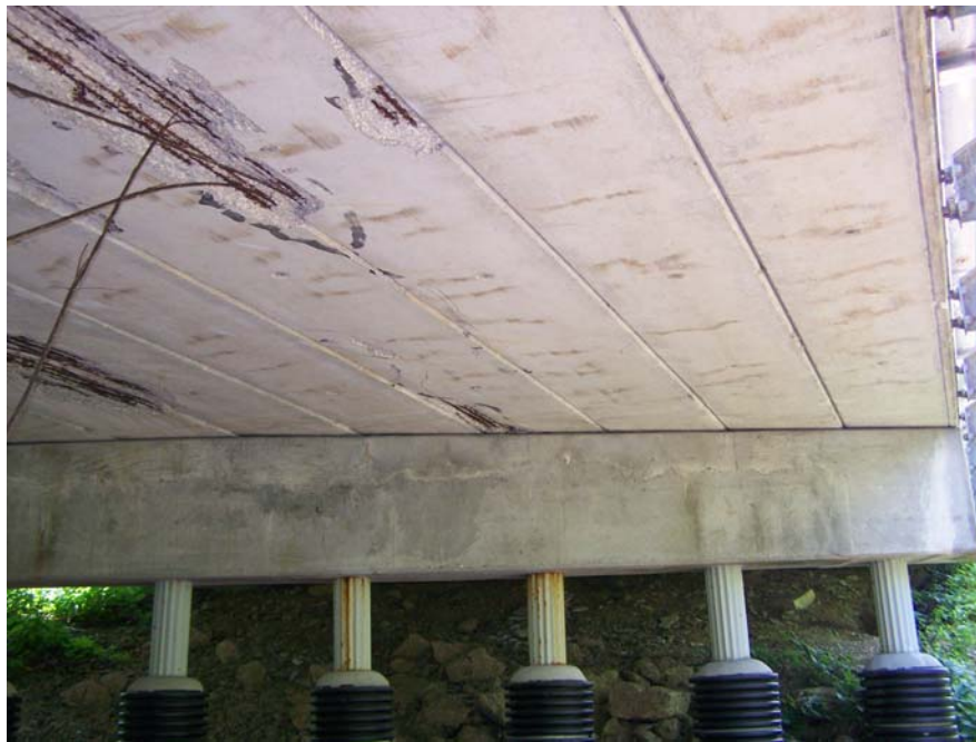
Fig. 3: Middle Span West Side
