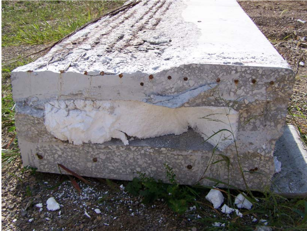
Fig. 12: Beam 18 North Section
