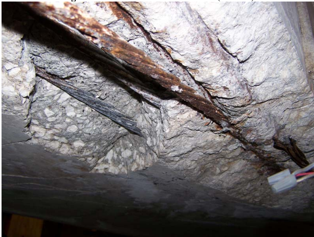
Fig. 15: Destructive Test of Beam 16 (Bottom)
