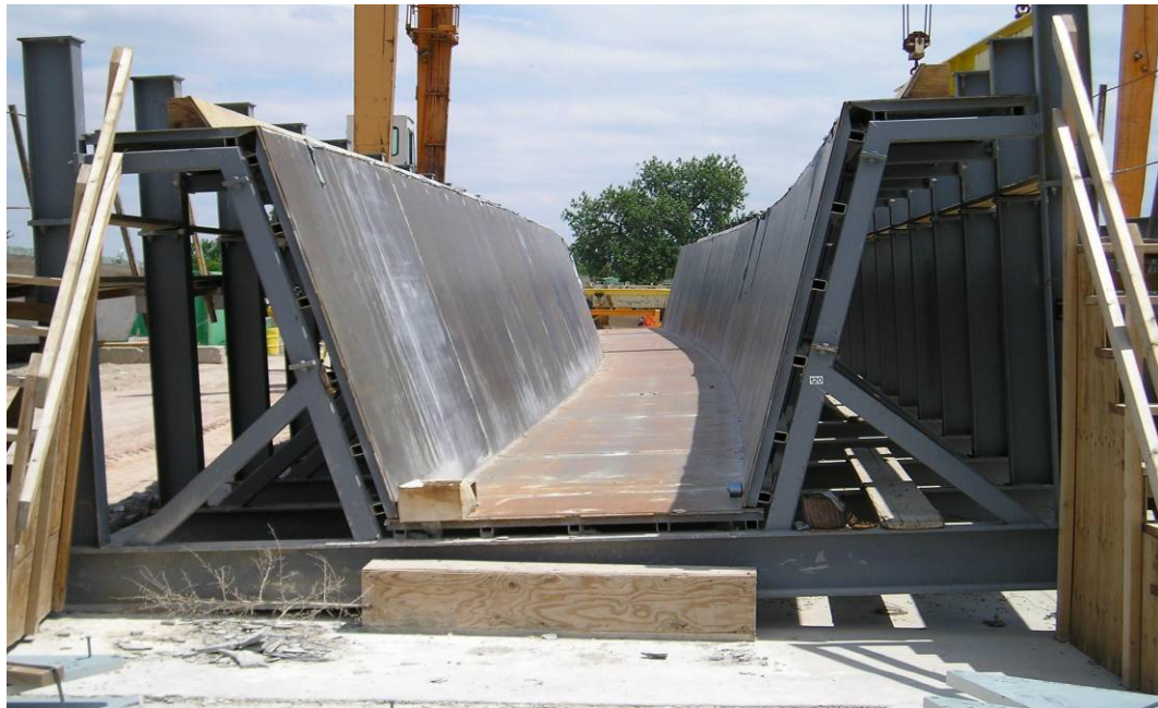
Fig. 5: Precast U Girder Curved Forms
