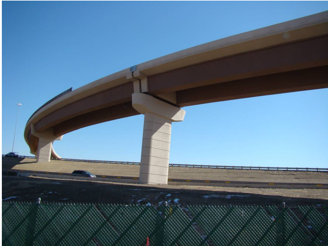
Fig. 4: Ramp A, Expansion and Interior Piers
