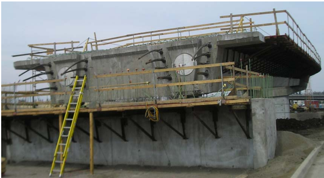
Fig. 11: Cast-in-place End Diaphragm at Abutment 1
