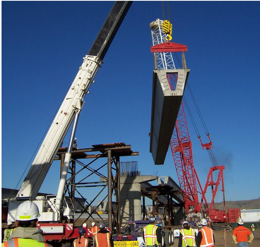
Fig. 9: Precast Girders Set on Falsework with Cranes
