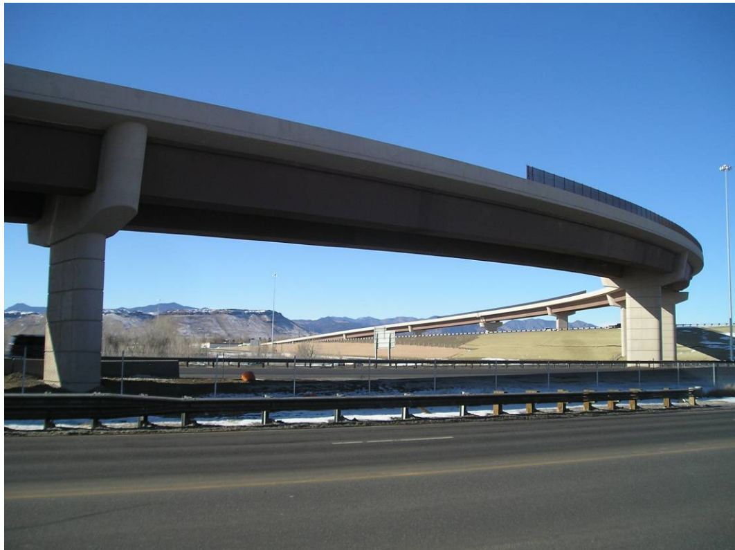
Fig. 1: SH58 Ramp A Bridge
