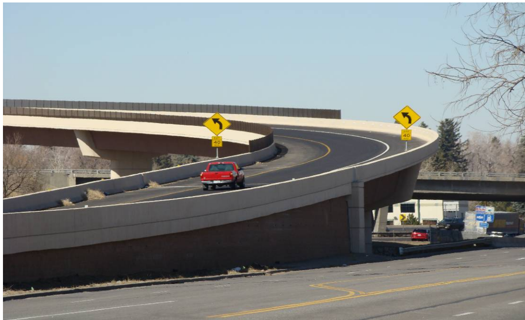
Fig. 2: Abutment 1 access to SH58 Ramp A Bridge
