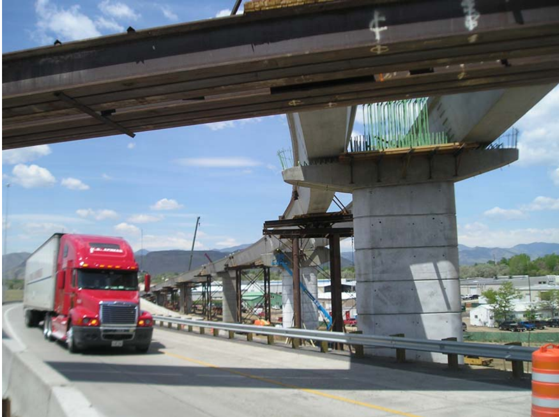
Fig. 10: Precast Girders Set on Straddle Bent and Falsework at Traffic Opening
