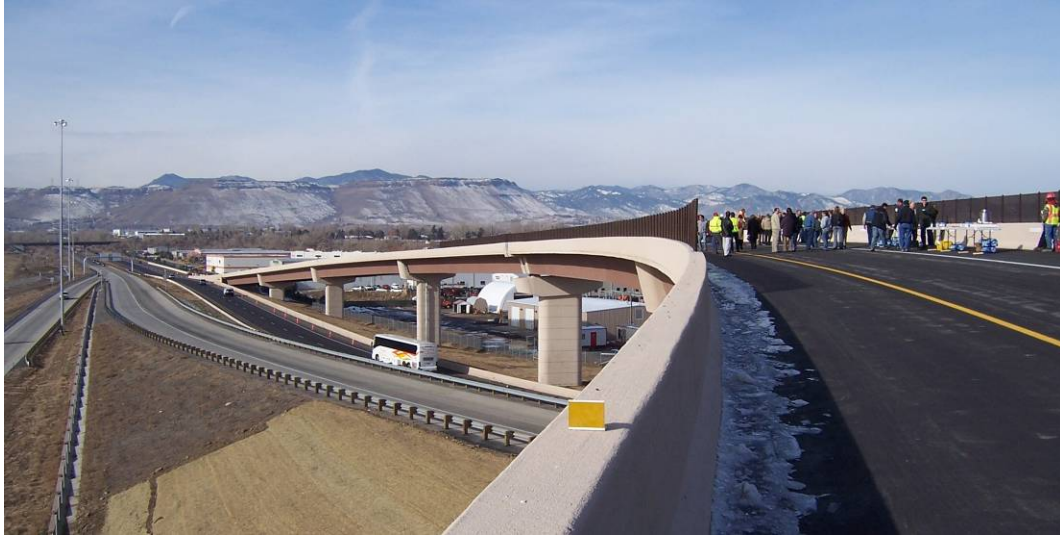
Fig. 3: Ramp A, Units 2 & 3 at Abutment 12
