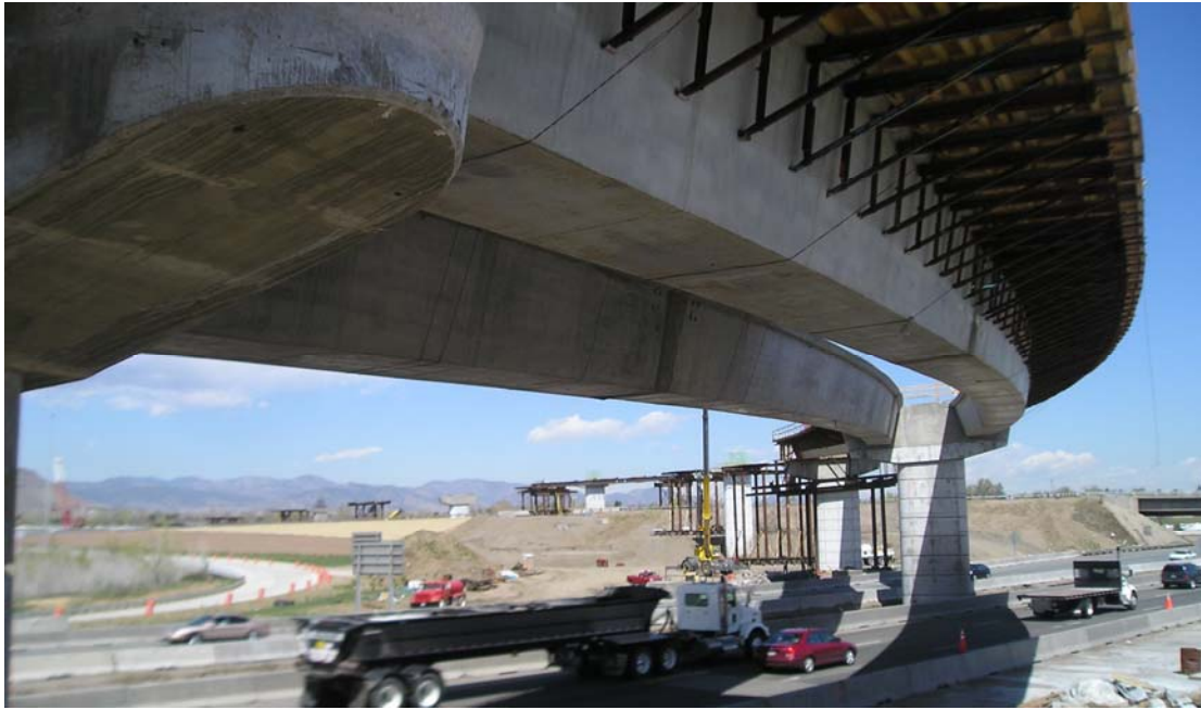
Fig. 12: Shoring is Removed after Post-tensioning before Casting Deck Slab
