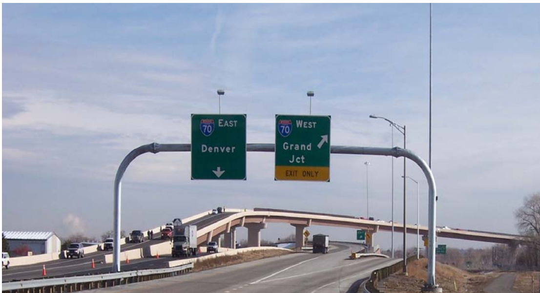
Fig. 13: Ramp A Opened to Traffic, November 2008
