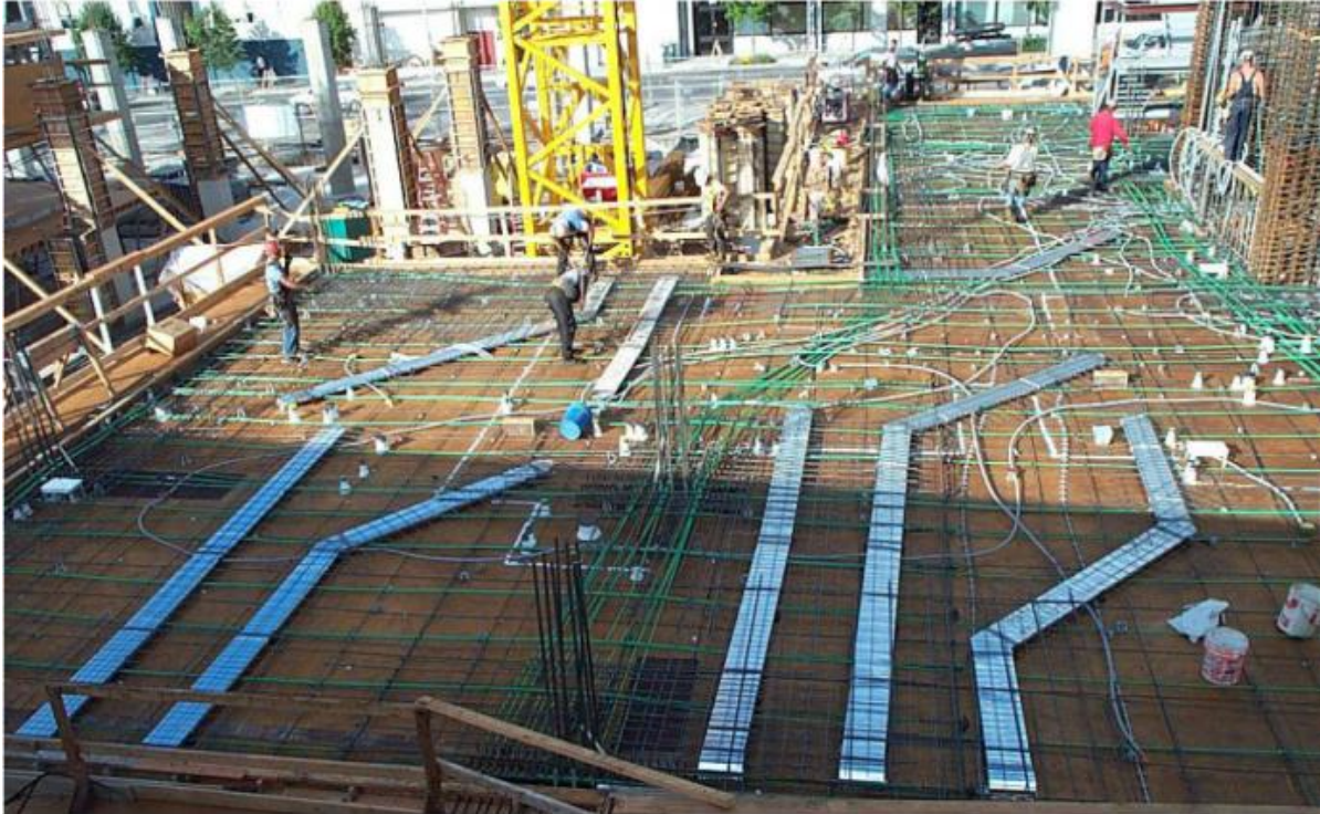
Fig. 1 Construction of post-tensioned cast-in-place concrete slab (PTI 2006)
