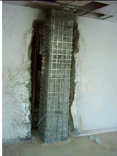
Fig. 5 Grouting and zinc mesh installation
