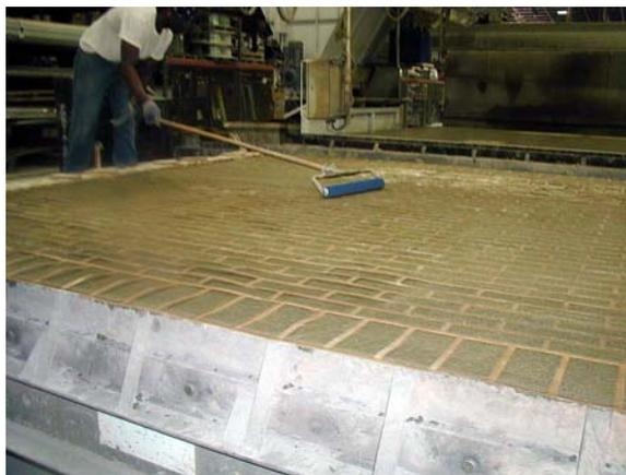
Fig. 9. A texture roller is used to embed stencils
