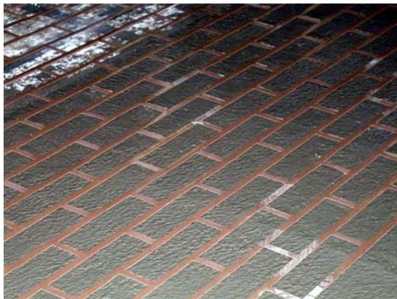
Fig. 10. Stencils are embedded flush with the concrete surface
