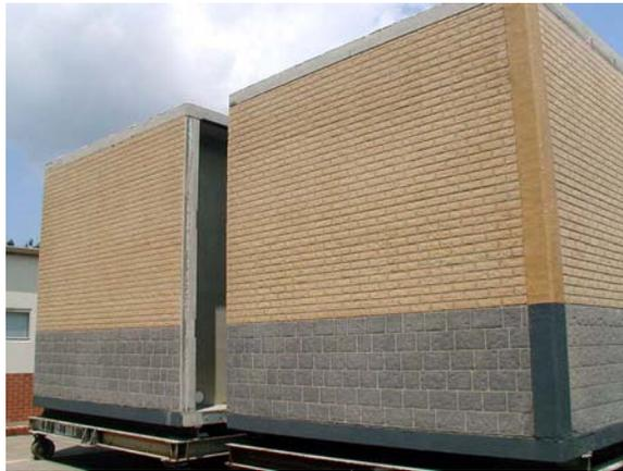
Fig. 17. Completed stencil-finished precast concrete panels
