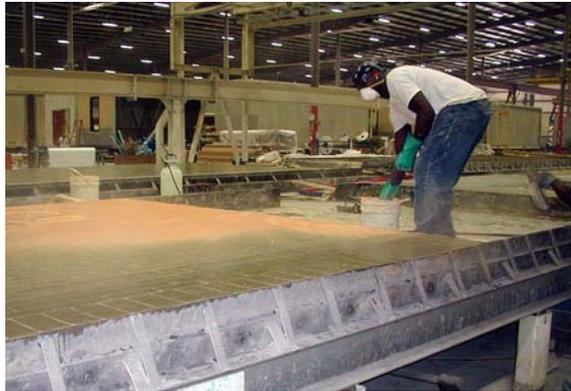
Fig. 11. Color hardener is broadcast onto concrete
