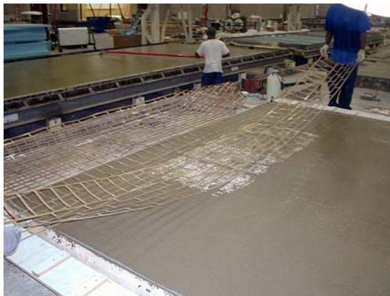
Fig. 6. Stencils are placed across the width of the precast concrete panel
