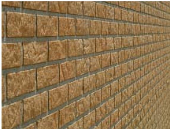
Fig. 18. Stencil-finished precast concrete panel texture
