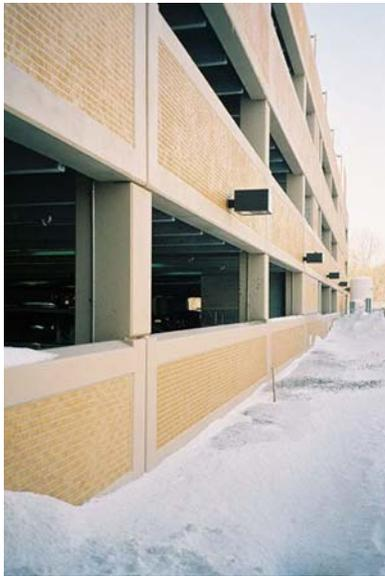
Fig. 22. Example of a parking garage utilizing stencil-finished precast concrete panels
