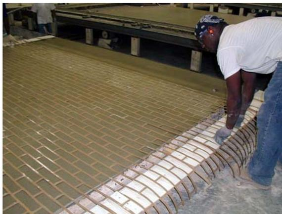
Fig. 7. Stencils are overlapped for pattern continuity
