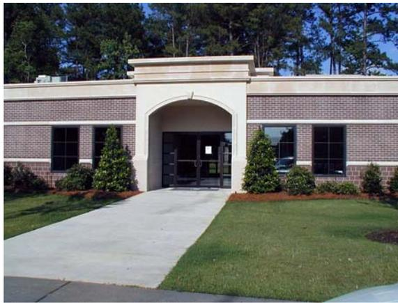
Fig. 19. Example project utilizing stencil-finished precast concrete panels
