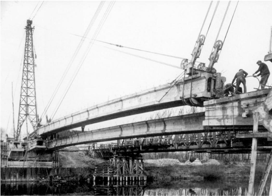
Figure 11 - Luzancy Bridge segment erection
