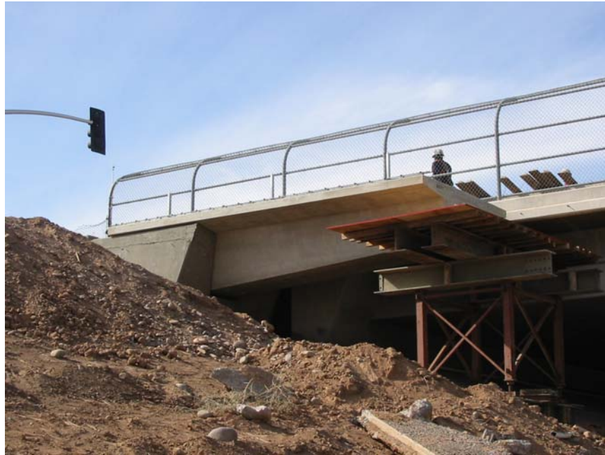
Figure 9: Falsework at End Segment
