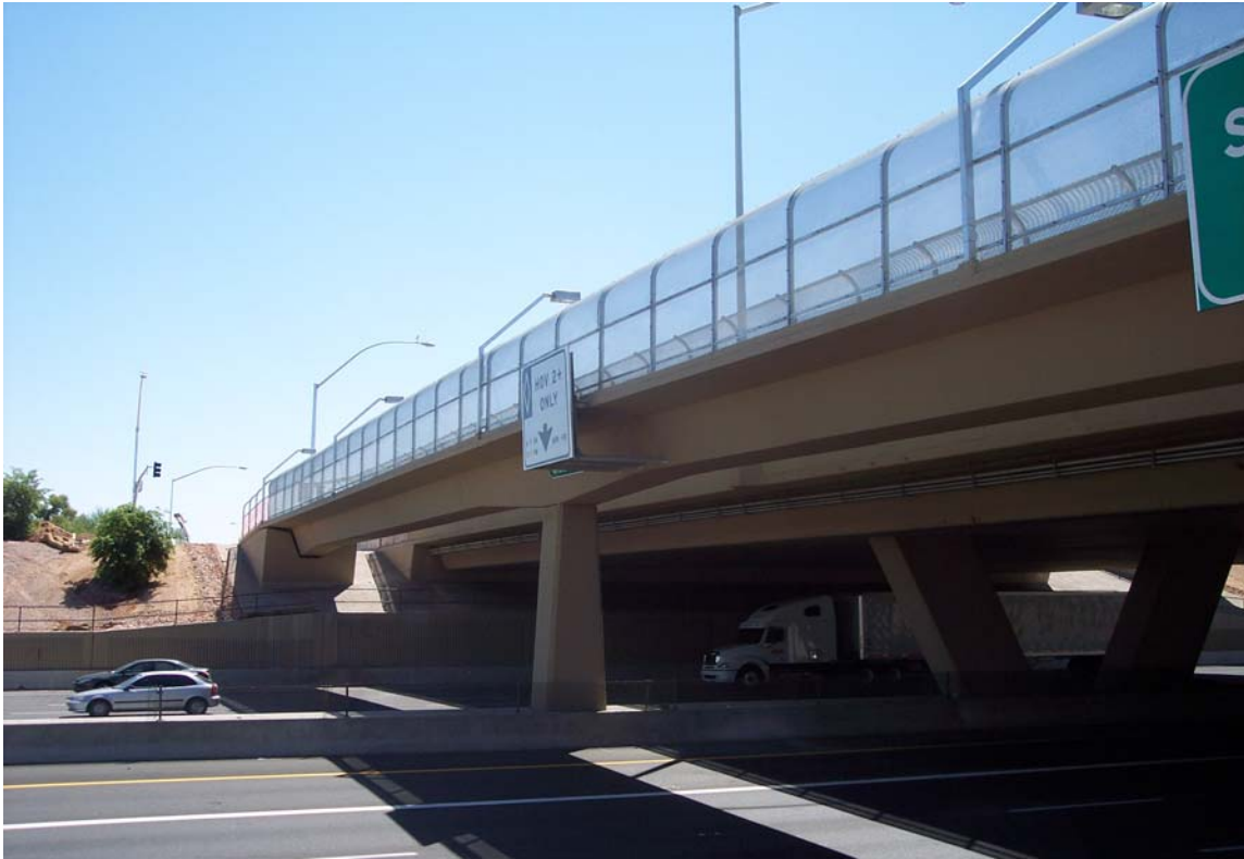
Figure 15: Completed Bridge at Rural Road
