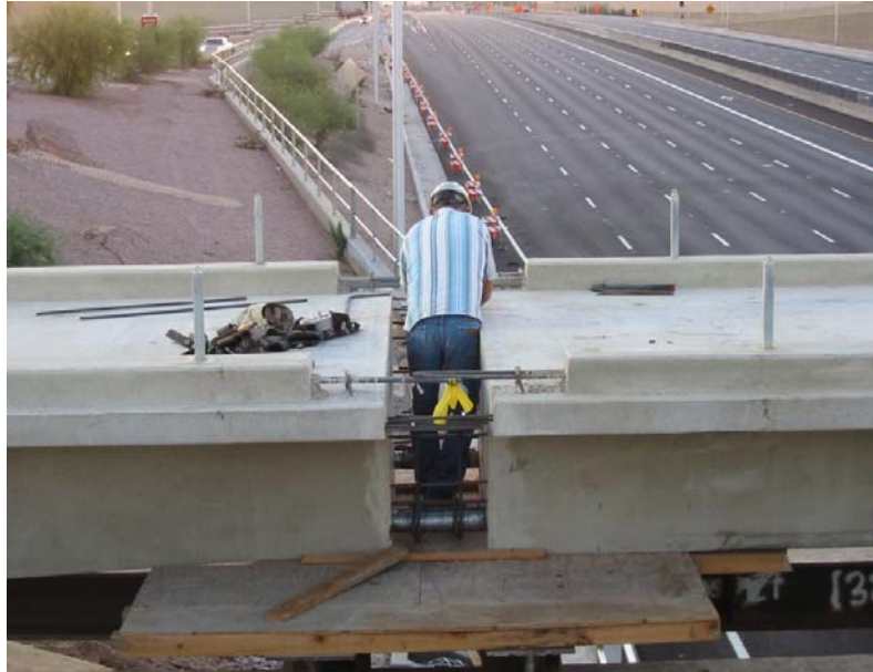
Figure 12: Preparing the Closure for Grouting
