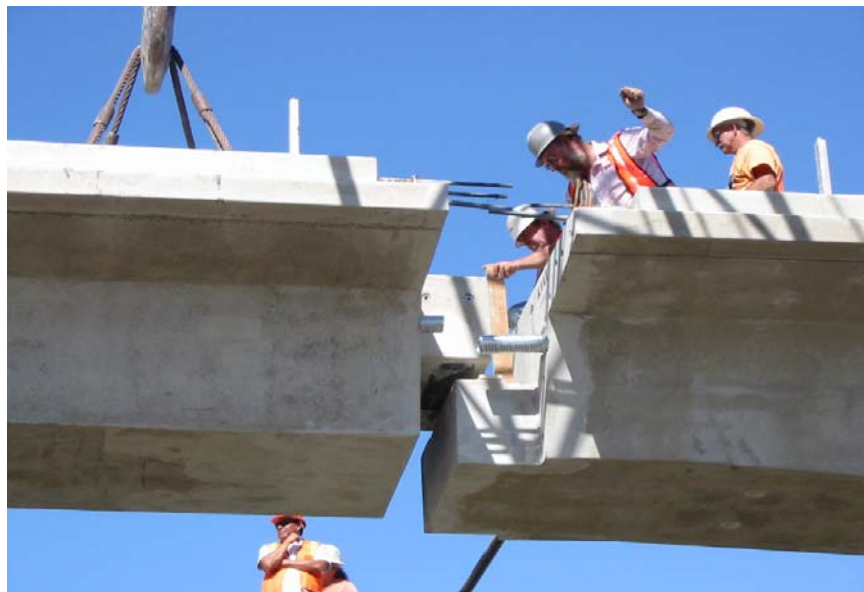
Figure 11: Setting the Drop-In Segment
