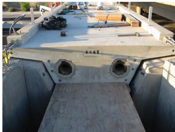
Figure 13: Abutment Segment Prior to Post-Tensioning
