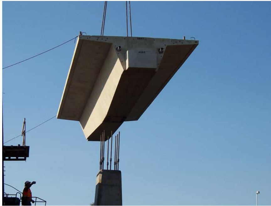
Figure 10: Erecting the Pier Segment
