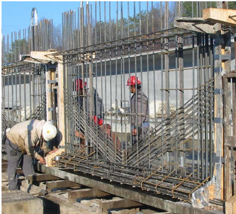
Figure 6. BT-72 mock-up beams with 42 0.6-in. strands.
