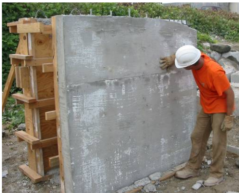
Figure 1. 6-in. thick wall panel
