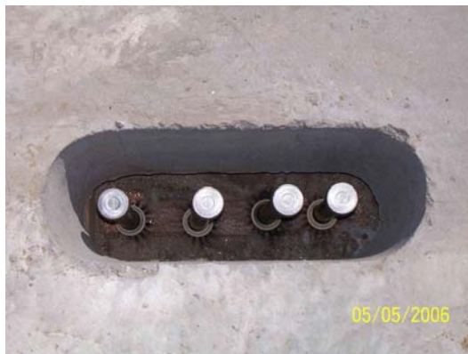
Fig. 13 Shear Connectors
