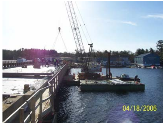
Fig. 7 Panel Erection From Barge
