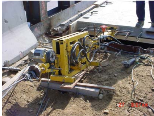
Fig. 9 Hydraulic Strand Feeder
