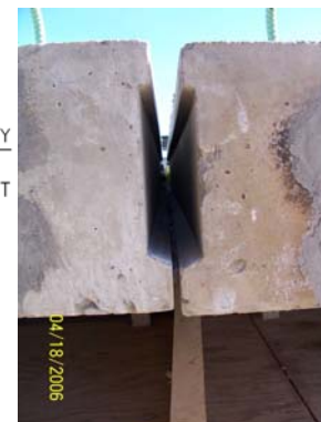
Fig. 4 Shear Key
