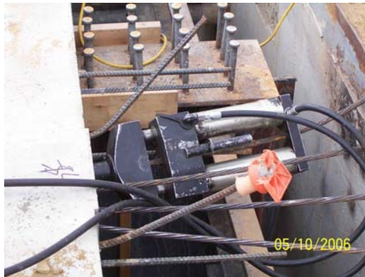
Fig. 12 Jacking of Post Tensioning
