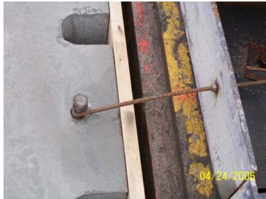
Fig. 6 Blockout along Middle Girder
