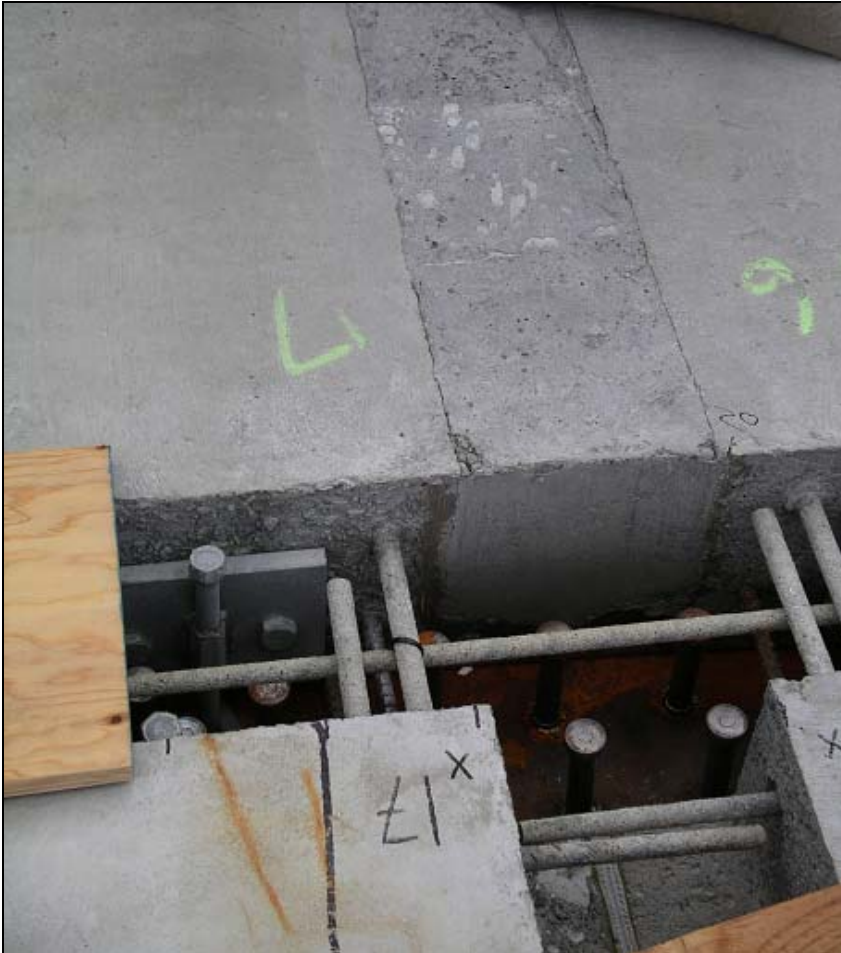
Fig. 8 Joints ready for filling with UHPC
