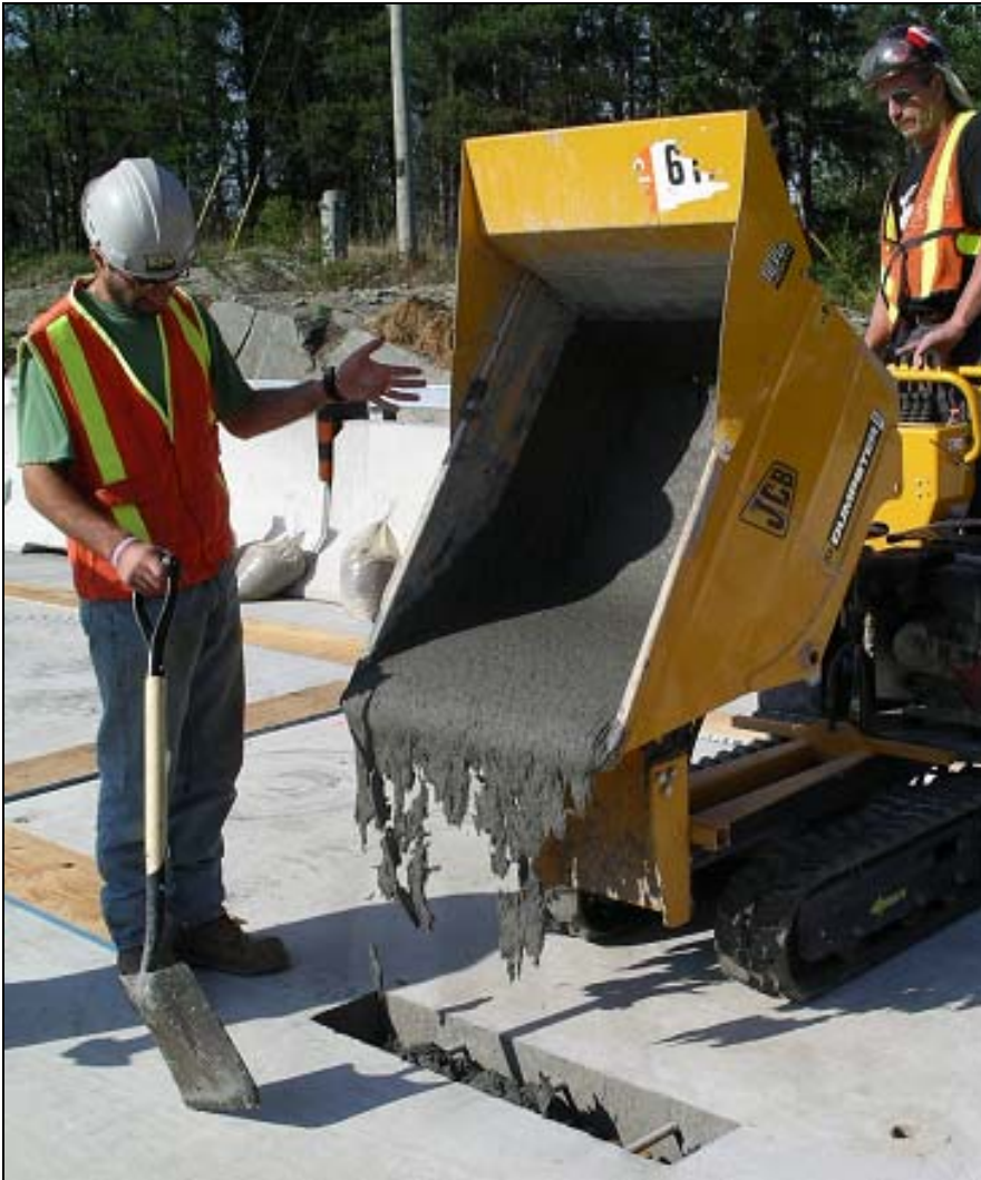
Fig. 9 Filling the joints with UHPC placed from the power buggy
