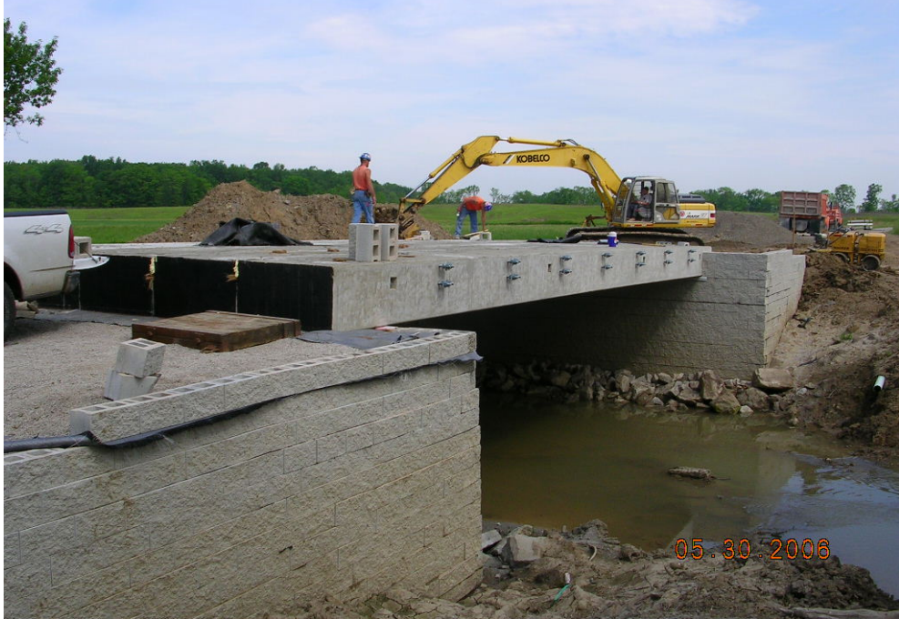
Figure 10. Placement of Beams on GRS Abutment for the Glenberg Bridge
