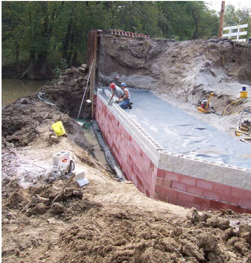
Figure 7. Construction of GRS Abutment
