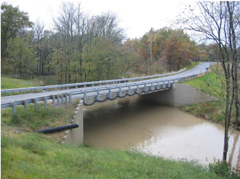
Figure 13. Completed Bowman Road Bridge
