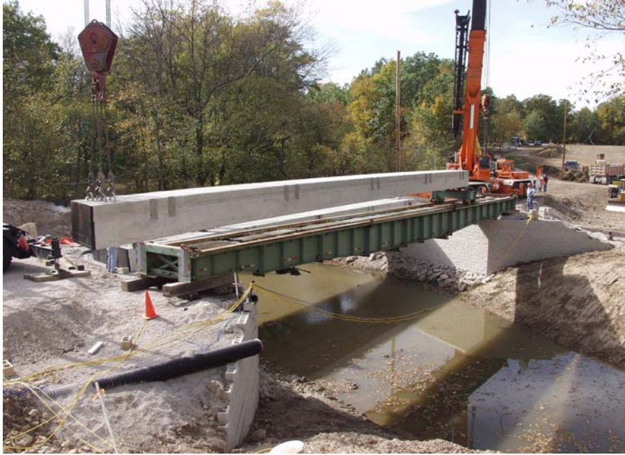
Figure 8. Placement of Concrete Box Beam on GRS Abutment
