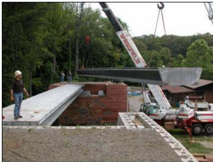
Fig. 10 Installing pi-girders at the FHWA Turner-Fairbank Laboratory
