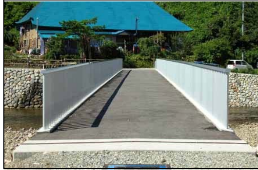
Fig. 6 The Yokemuri Footbridge in Yamagata, Japan
