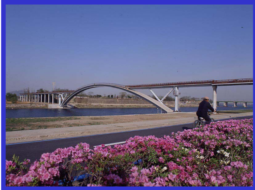
Fig. 4 The Seonyu Footbridge in Seoul, Korea
