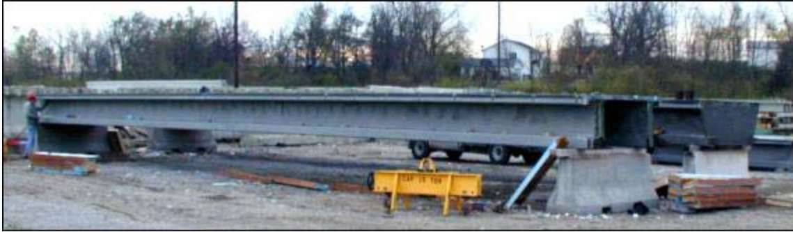
Fig. 9a Pi-girders at Prestress Service, Lexington, KY
