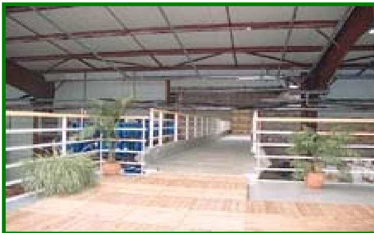
Figure 3 – Footbridge in Chryso Plant, Sermaise, France
