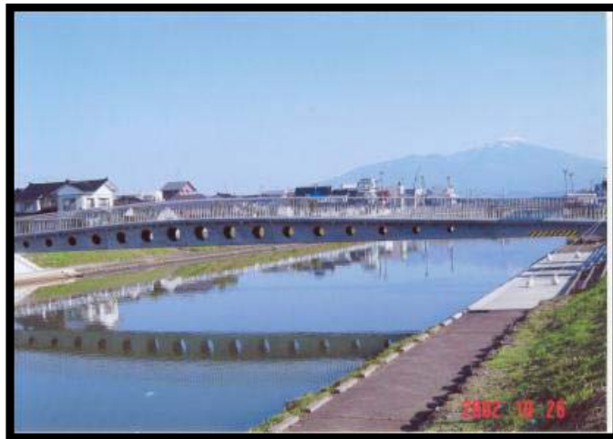
Fig. 5 The Sakata Mirai Footbridge in Sakata, Japan
