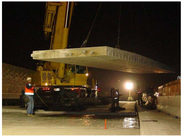
Installation of precast panels for the California demonstration project.
