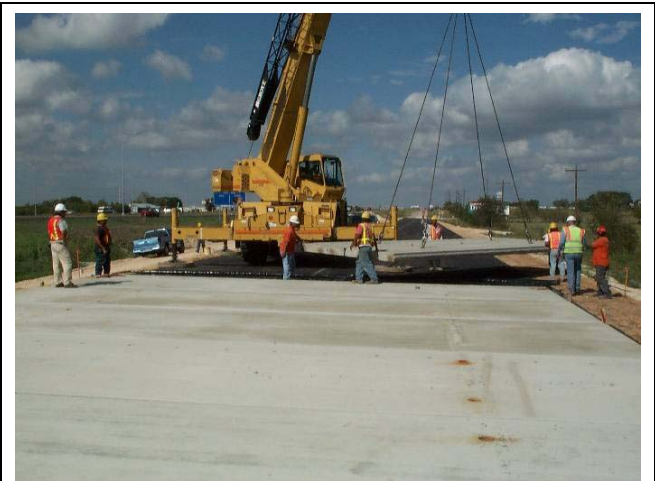
Installation of precast panels for the Georgetown, Texas pilot project.
