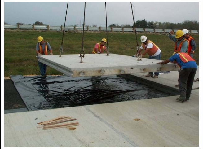
Installation of precast panels for the Georgetown, Texas pilot project.
