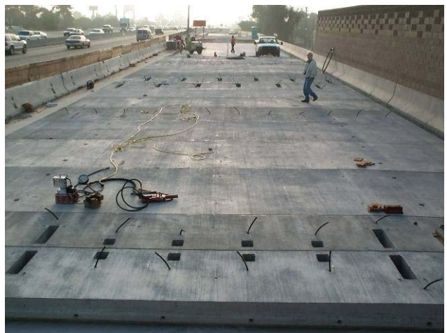
Installation of precast panels for the California demonstration project.
