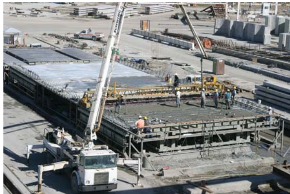
Figure 3 Precasting Double Tee Girder
