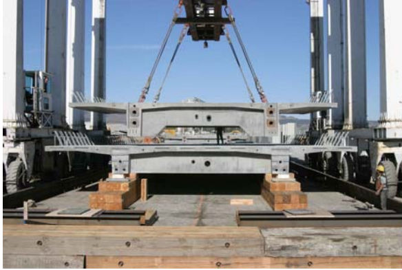
Figure 4 Loading Girder Segments on Barge
