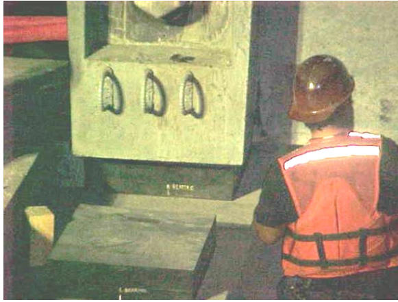
Figure 12 Girder Joint Reinforcement
