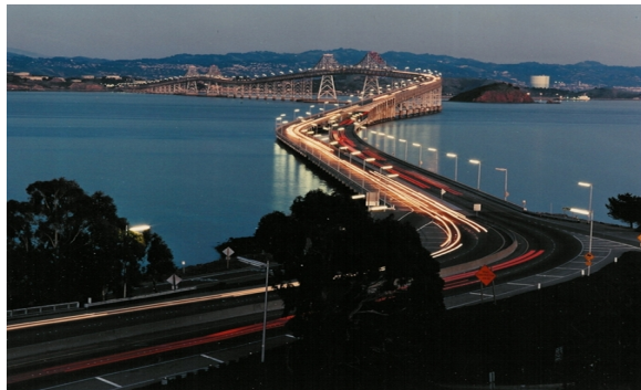
Figure 1 Richmond San Rafael Bridge
