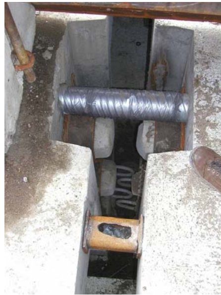
Figure 13 Closure Joint Ready for Pour
