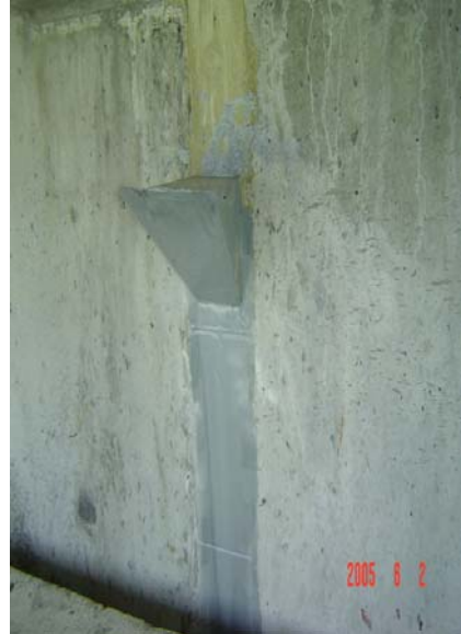
Figure 19 Second Stage Closure Pour with Elastomeric Concrete
