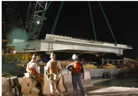
Figure 6 Lifting New 100-Foot Span
