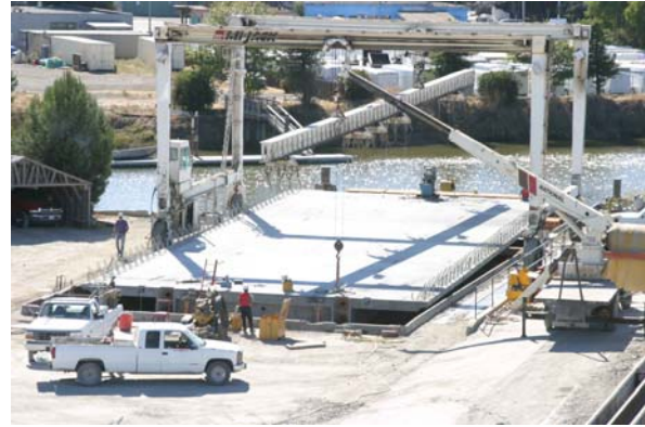
Figure 5 Post Tensioning on Barge
