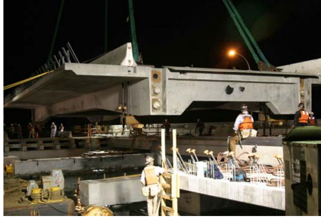
Figure 7 Placement of 100-Foot End Span
