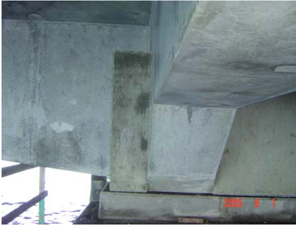
Figure 18 Completed Closure Joint Bolster
