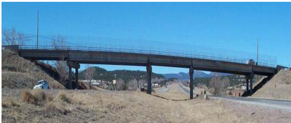
Figure 1 - Photo of Old Bridge
