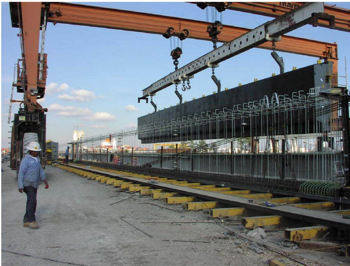
Figure 2. Construction of 145 ft. long by 95.5 in. deep Bulb-T for Unit B
