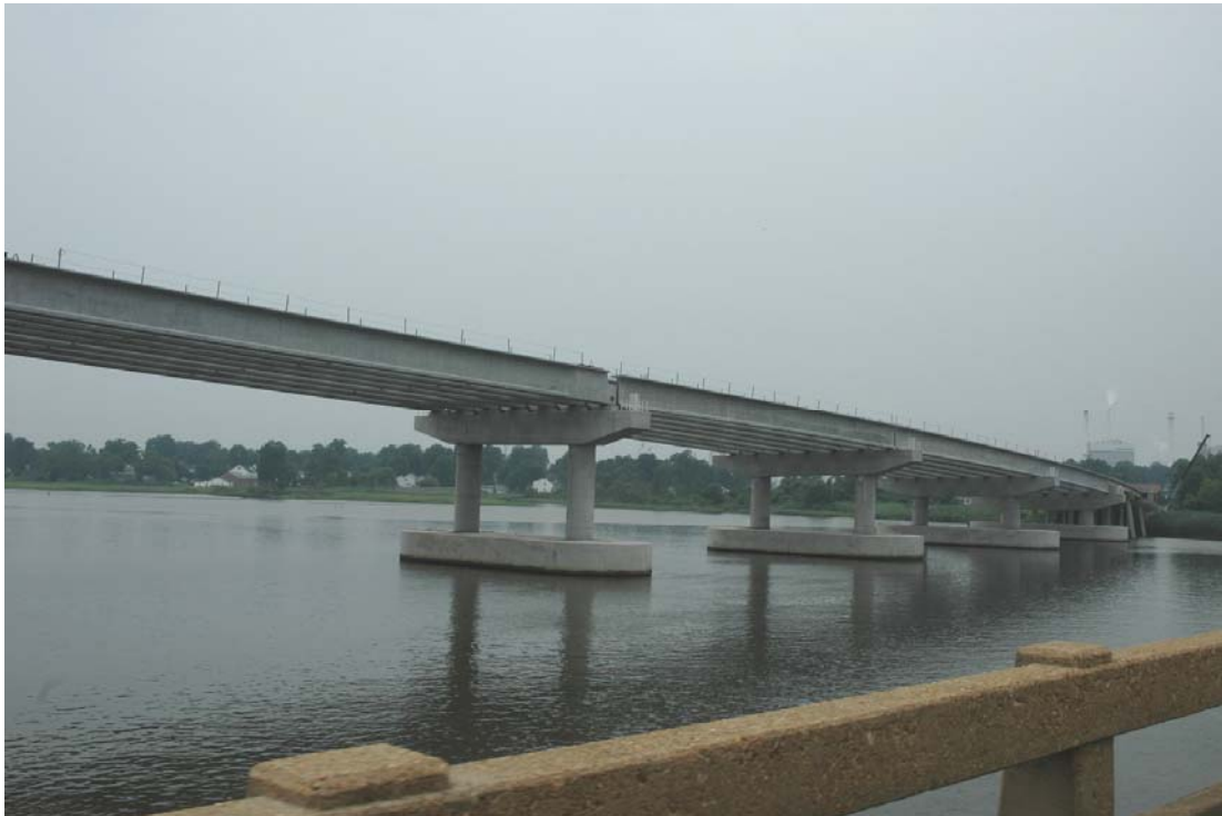
Figure 1. Unit B 3-span approach from West Point to splice girder channel span units.
