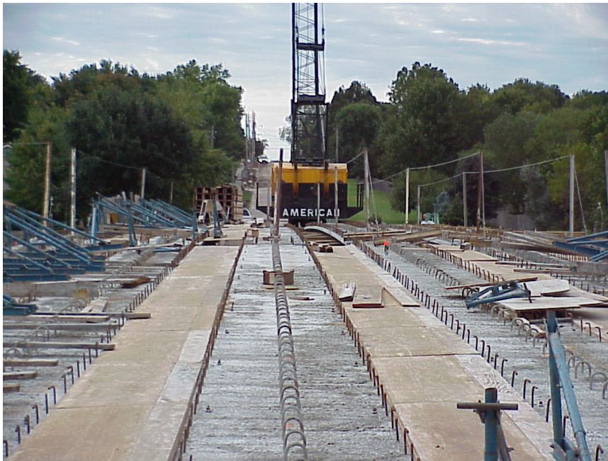
Figure 9 (Formwork in Place 28 th St.)
