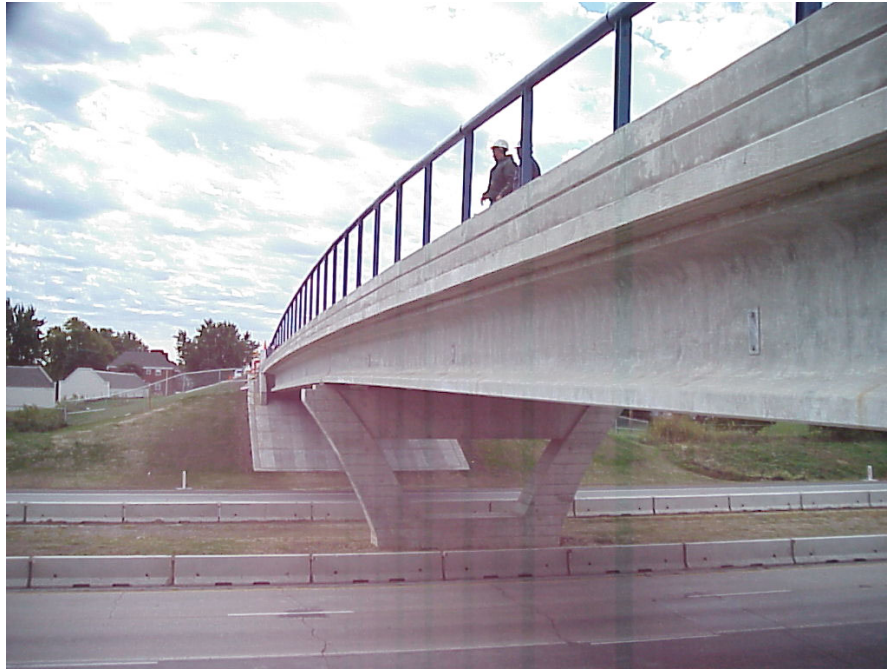
Figure 10 (Completed 28 th St. Bridge)
