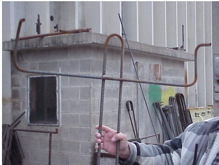
Figure No. 11 (Top Flange Reinforcing Detail)
