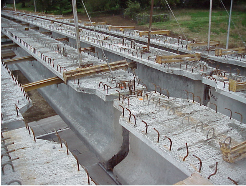
Figure 8 (Beams Erected 28 th St.)
