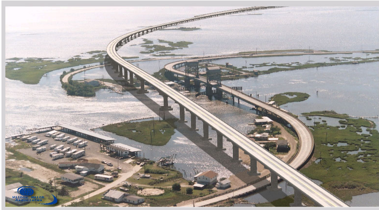
Three Span Channel Unit at Leeville, LA. 350 ft. Channel Span
