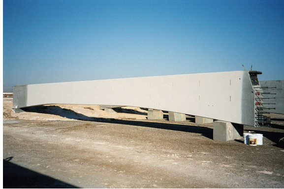
Fig. 4 LVMR, Rails in the casting yard
