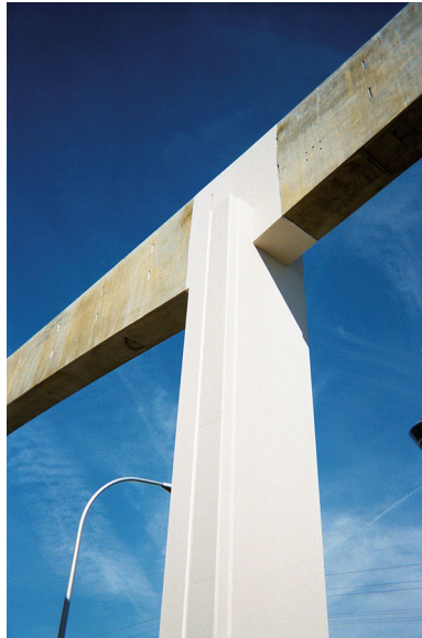
Fig. 3 Stained pylon meets unstained rail sections
