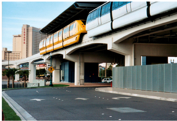
Fig. 2 Completed section of the Las Vegas Monorail
