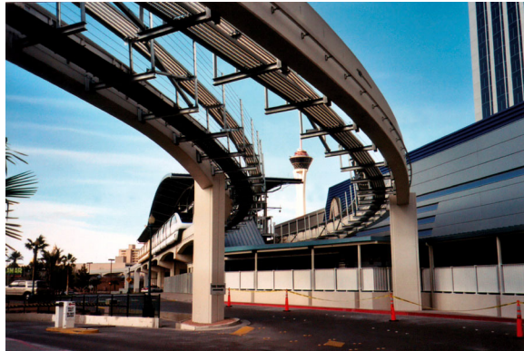
Fig. 1 Los Vegas Monorail nears completion
